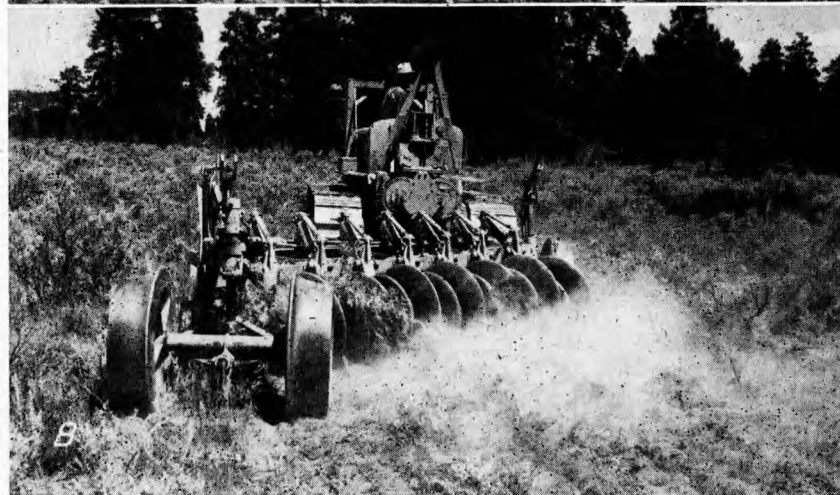
FIGURE 12.—The brushland plow: A, This plow is killing the low-value vegetation, the cultipacker is firming the seedbed, and the seed is being drilled in one operation, at a cost of $2.50 per acre, exclusive of seed; B, this brushland plow is doing a good job of killing sagebrush in the ponderosa pine zone.
