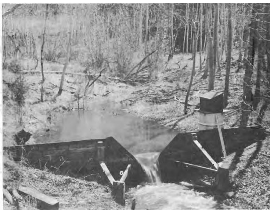
Figure 10. 90° V-notch weir installed in North Fork of Missouri Gulch. From Berndt (1960).
