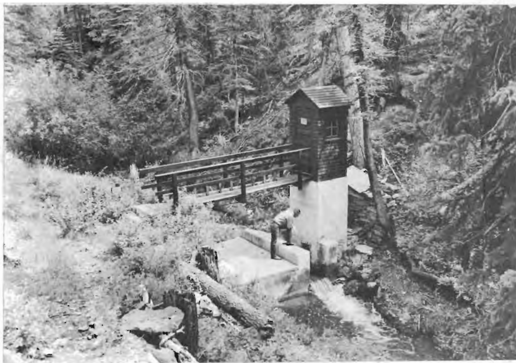
Figure 9. San Vitas Flume installed near the mouth of the Missouri Gulch watershed. From Berndt (1960).
