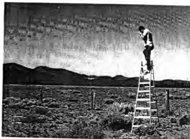
FIGURE 2.—Near-vertical ground photographs of marked targets are taken on or near the day of the photo mission, and make up a vital part of the ground truth. Note low-flying photo plane.
