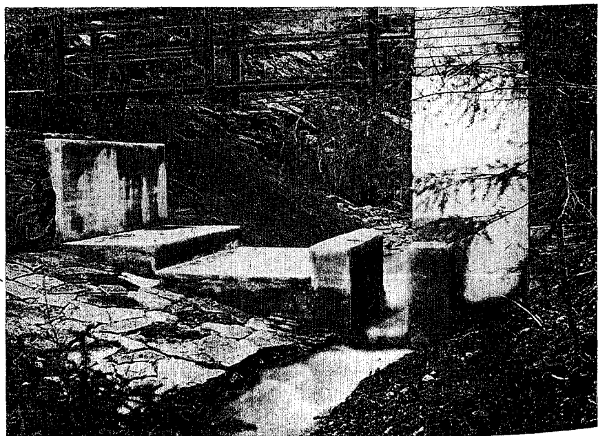
GAGING STATION IN MANITOU EXPERIMENTAL FOREST, COLORADO, FROM DOWNSTREAM Normal Flow Measured in 2-Ft Flume, Peak Discharges Over One or Both of Adjacent Broad-Crested Weirs
