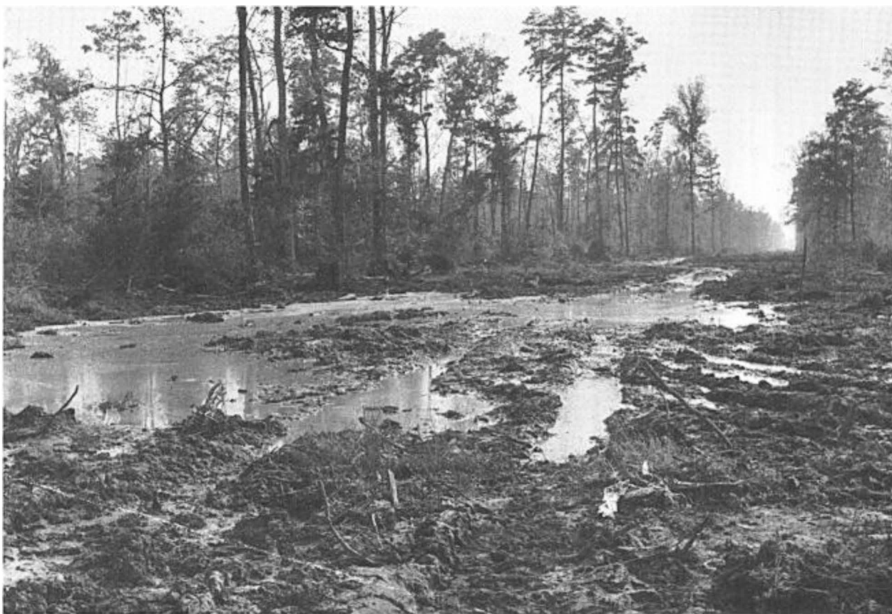
Clearing prior to construction of drainage ditch. Photo courtesy Westvaco Corporation.
