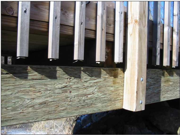
Figure 13. Pressure-treated parallel strand lumber (PSL) beams were used as supports for this trail bridge.
