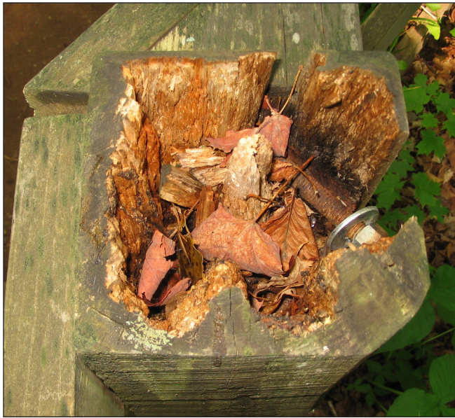
Figure 25. Sawn posts may contain poorly treated heartwood that is exposed if the post is cut to height after installation. If cutting to height is necessary, the exposed top should be coated with a field treatment preservative such as copper naphthenate.
