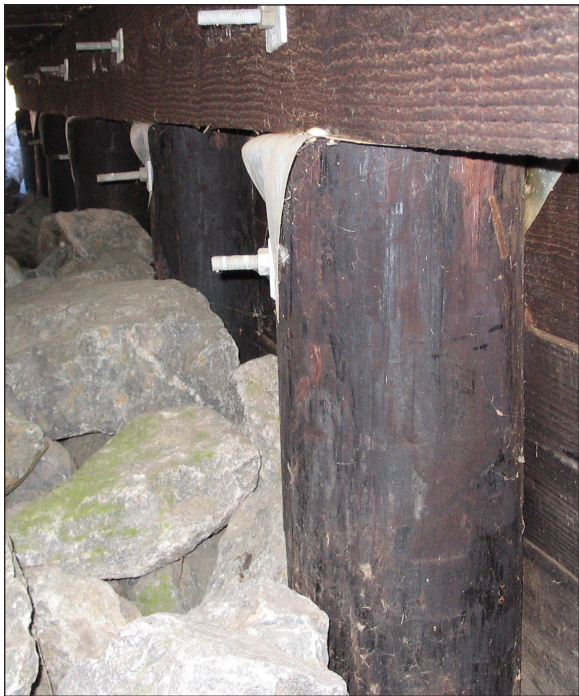
Figure 11. Pressure-treated round support piles used in applications such as this highway bridge are structurally critical and have a high decay hazard. They are treated to meet AWPA Use Category 4C.
