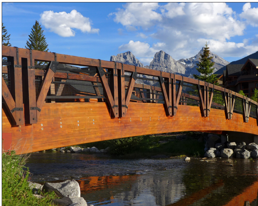
Figure 12. Pressure-treated glue-laminated timbers are frequently used to support bridges and in other applications with long spans and/or high strength requirements
