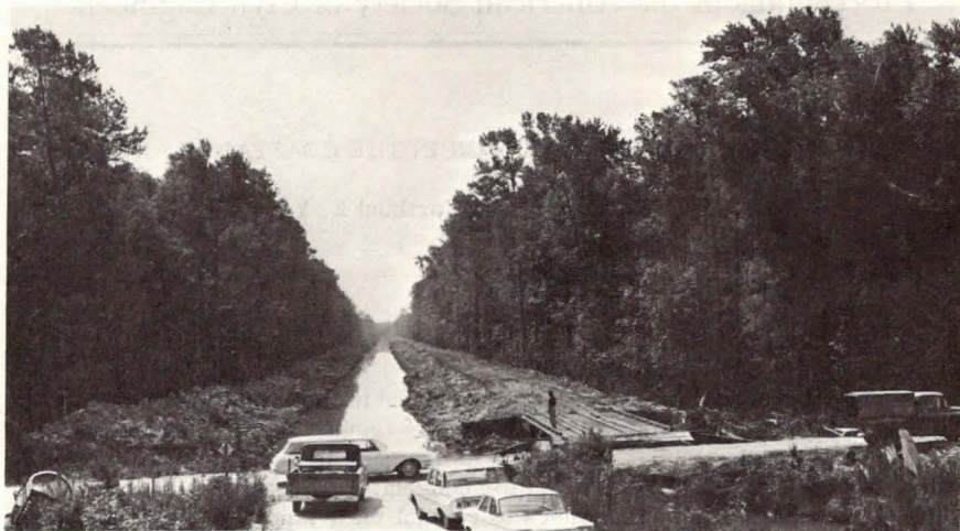
FIG. 1.—NEWLY CONSTRUCTED ACCESS ROAD AND DITCH INTO LARGE, UNDEVELOPED TRACT OF WETLAND FOREST
