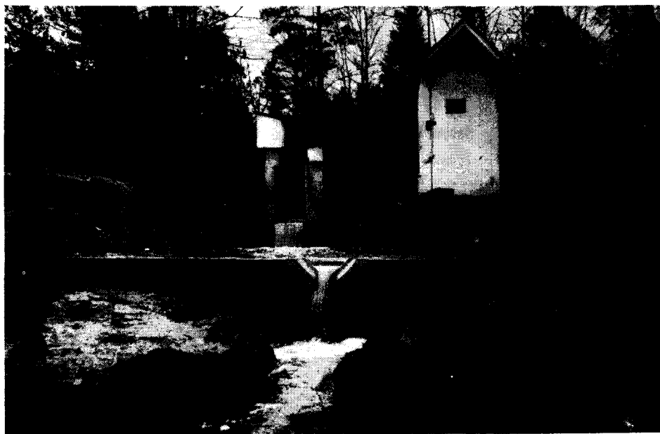
This installation on the Calhoun Experimental Forest measures runoff from a small watershed as part of a program to determine measures needed to improve the water resource
