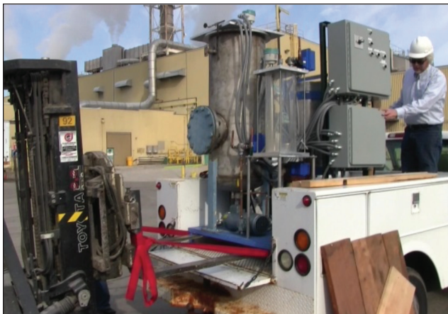
9. Pilot unit being unloaded.
