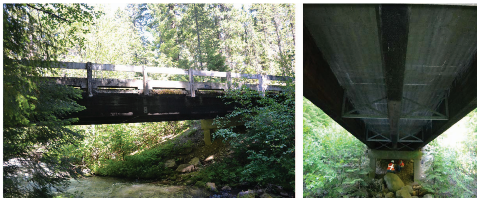
Fig. 5. (Color) T-deck glued laminated bridge in Gifford Pinchot National Forest (Salmon River Bridge). (Images by Alfredo M. P. G. Dias.)
