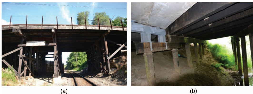
Fig. 3. (Color) (a) Bridge built in 1901 in Illinois; and (b) bridge where new concrete members were added to an original timber beam bridge. (Images by Alfredo M. P. G. Dias.)
