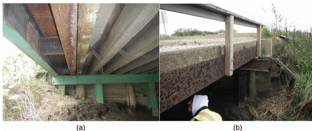
Fig. 14. (Color) (a) Widening; and (b) reinforcement of TCC bridges. (Images by Alfredo M. P. G. Dias.)
