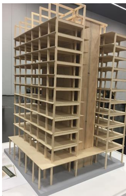
Figure 1. The building design with the cross-laminated timber (CLT) is a high-rise building structure in Portland, Oregon, USA.
