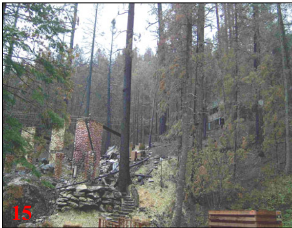
Photos 15,16—homes destroyed adjacent to homes survived indicates that significant differences existed in the fire and home characteristics necessary to meet the requirements for home ignition.
