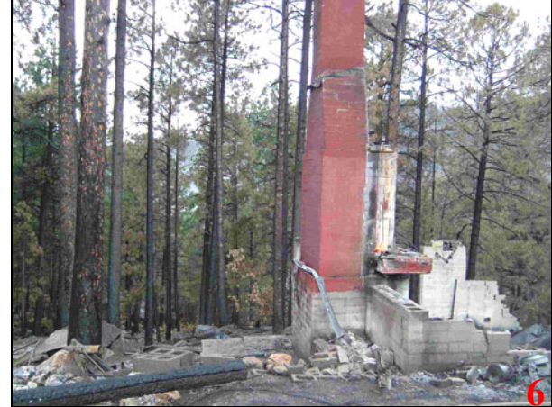
Photo 5,6—totally destroyed homes surrounded by unconsumed tree canopies indicate that lower intensity surface fires burned in the structures' surrounding areas.
