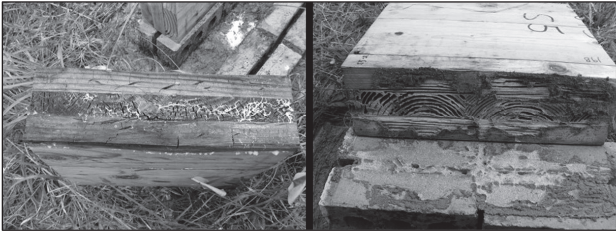
Figure 5. Examples of fungal decay (left) and termite (right) damage to 3-ply Douglas-fir CLT in a covered ground proximity test after two years.
