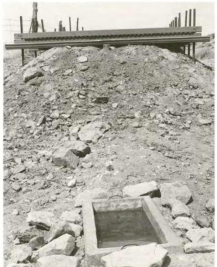
FIGURE 14. Precipitation catchments or "guzzlers" are of many designs but all can provide drinking water to range-land animals where no other possibilities exist (Sanderson et al. 1990).
