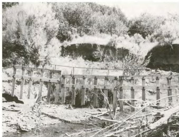
FIGURE 10. Swing gates across streams minimize maintenance following high water yet are effective as cattle barriers (Sanderson et al. 1990).
