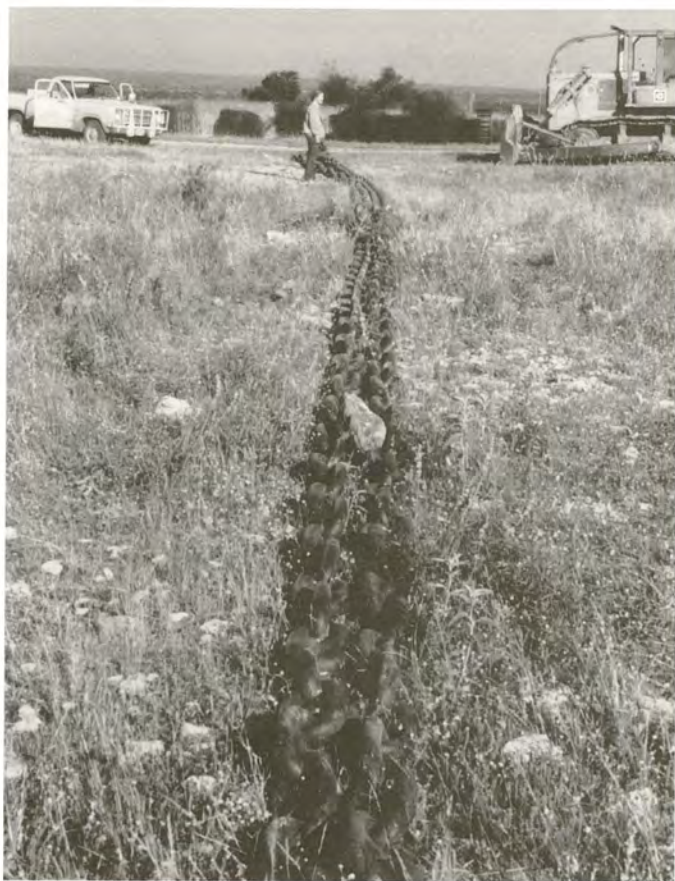
FIGURE 7. Anchor chain dragged between crawler tractors to uproot shrubs. Photo courtesy of Dale Rollins.
