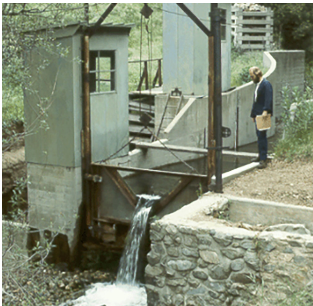
FIGURE 3 Gaging station at Volfe watershed. Note removable 90° v-notch weir in the throat of a 2.438 m (8 foot) San Dimas flume. (photo courtesy of Robert Lockwood)
