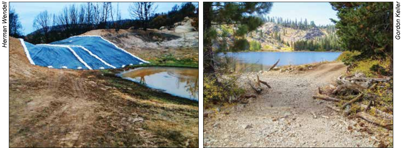
Figure 4.74—To prevent failure of old dams from overtopping or because of inoperable gate valves and structures, spillways of earth and rock are built or deepened.
