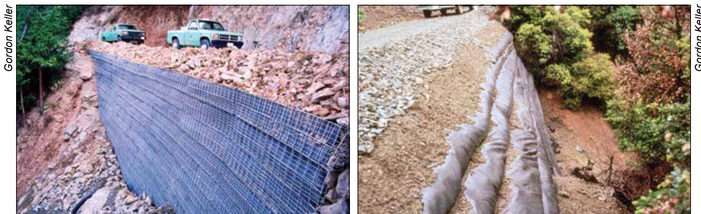
Figure 4.63—A welded wire, mechanically stabilized earth wall (left) and a geotextile wall (right) are both used because of their relatively low cost and ease of construction.
