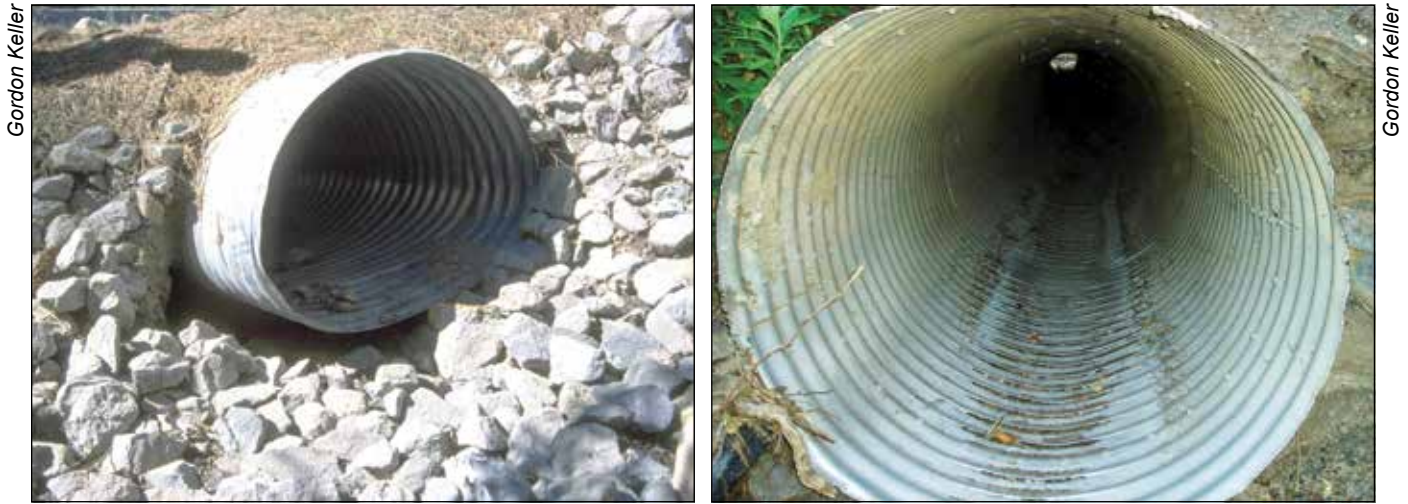
Figure 4.33—Problematic culverts owing to piping under the structure (left) or deterioration from a worn bottom (right). These culverts are at high risk of failure, particularly during major storms.
