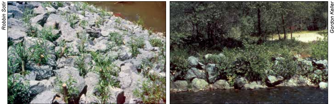
Figure 4.19—Biotechnical streambank stabilization using rock riprap and live willow stakes.
