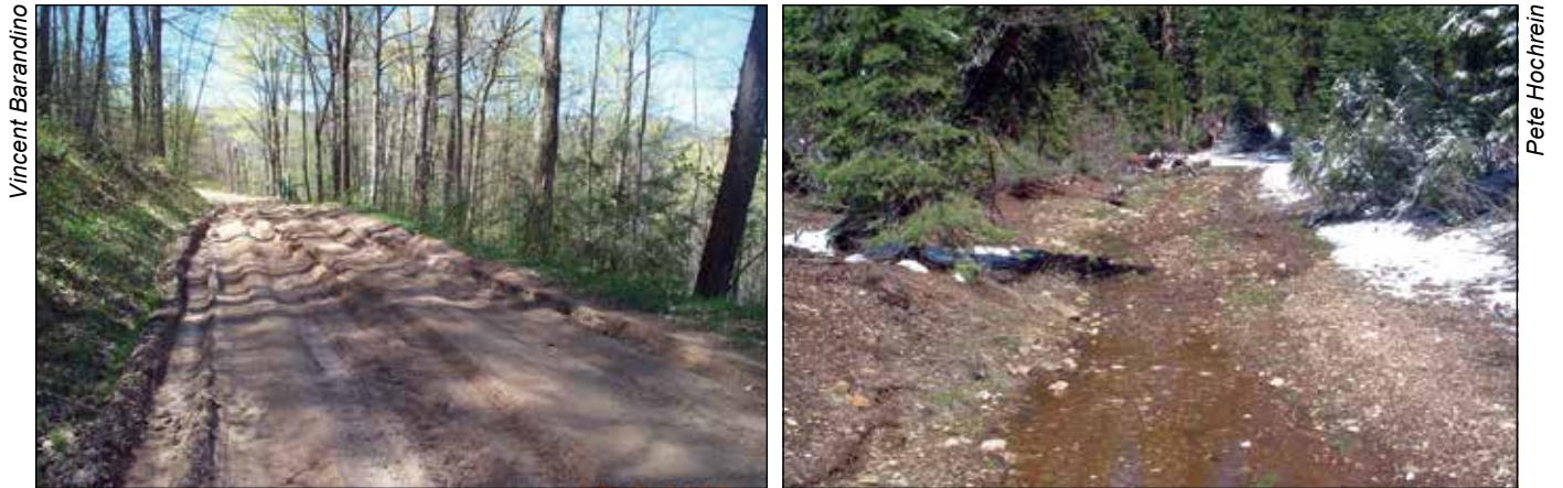
Figure 4.11—Ruts and erosion in the road surface because of lack of surface drainage and maintenance. Roads in this condition are particularly susceptible to storm damage.
