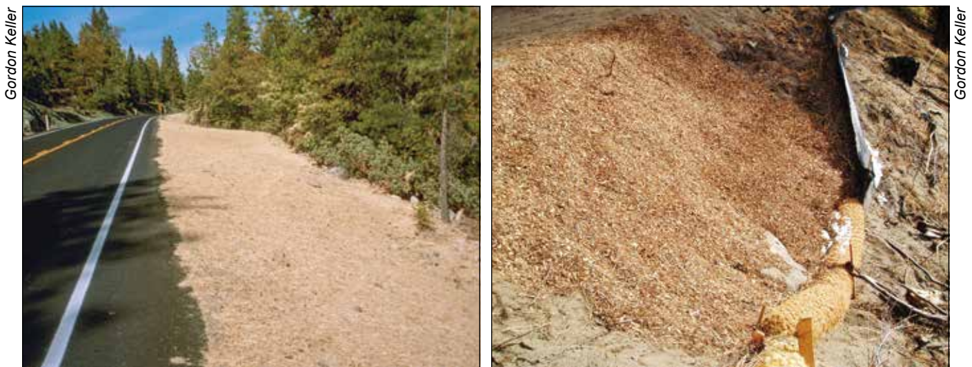
Figure 4.53—Common physical erosion control measures, including straw and netting (left), wood chips, and straw wattles (right), provide ground cover and surface stabilization until vegetation can grow.
