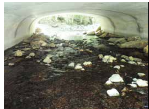
Figure 4.41—A stream simulation design through a culvert and a stream-simulation culvert installation. (Figure from Keller and Ketcheson [2015])
