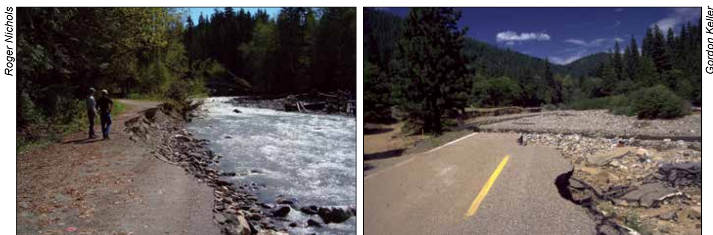
Figure 4.14—Roads located on the edge of a channel migration zone (left) and across a floodplain (right).
