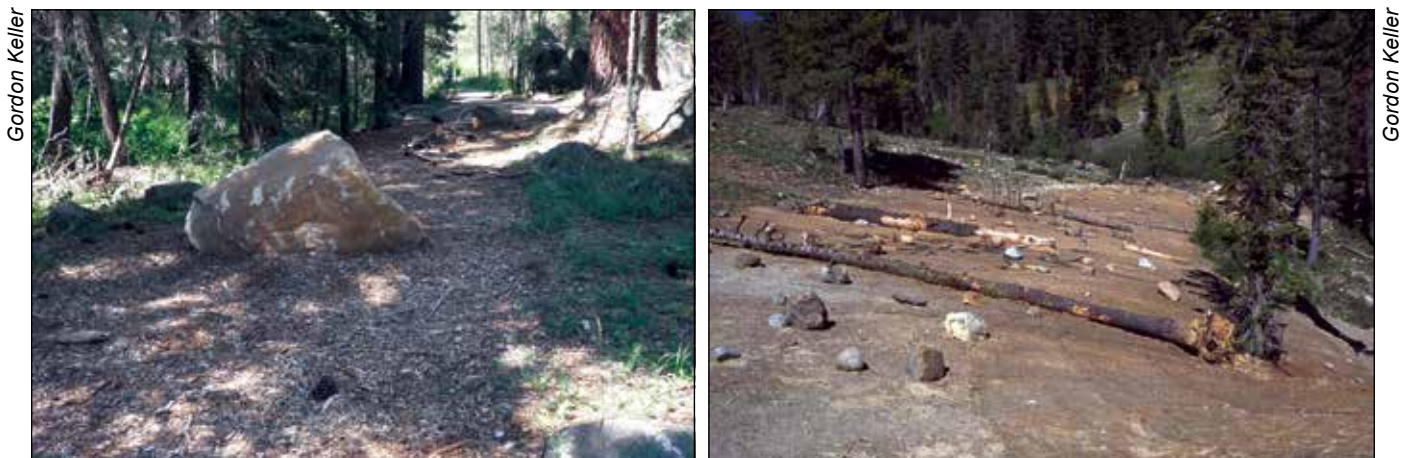
Figure 4.13—Road closure options include decommissioning (left) and complete roadway obliteration (right). Stormproofing with measures such as outsloping, frequent water bars or dips, and other treatments helps to ensure that maintenance is not needed to prevent damage.
