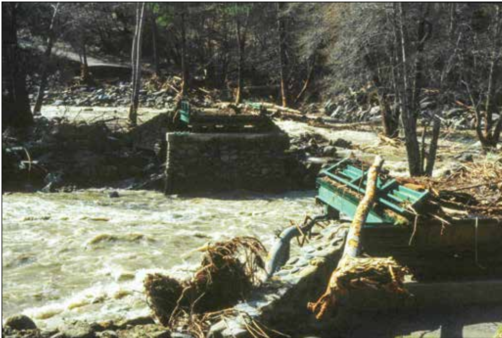
Figure 4.47—A failed bridge because of a lack of freeboard and accumulation of debris behind the bridge deck.
