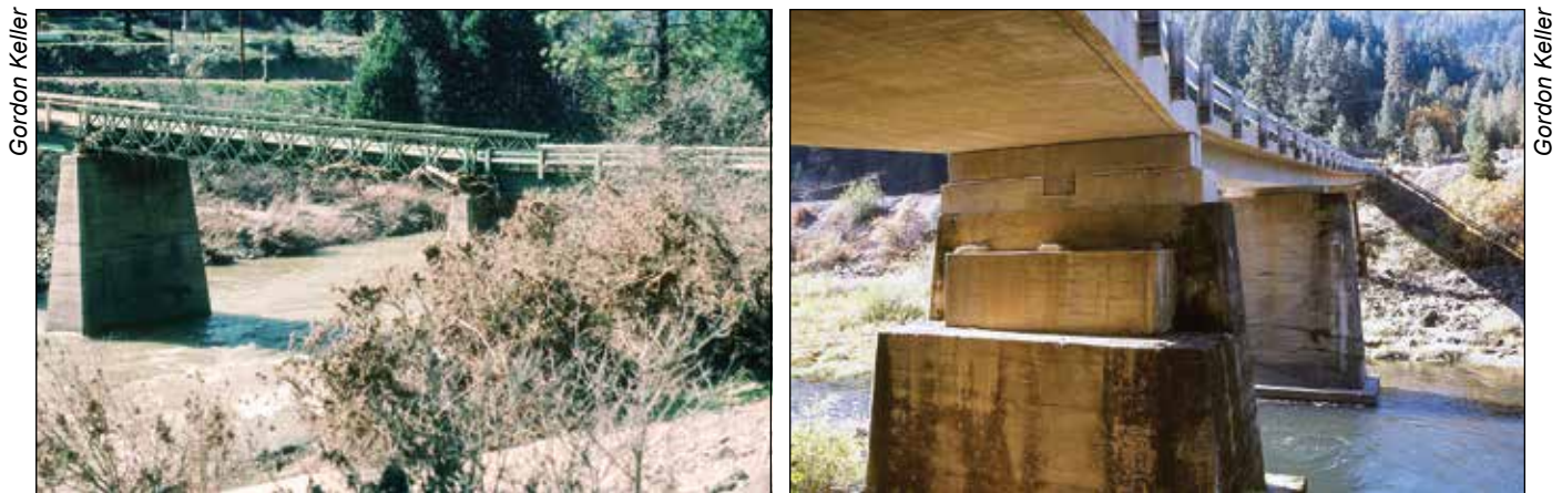
Figure 4.48—A bridge with marginal freeboard (left) whose abutments and piers were raised (right) to add freeboard and flow capacity.
