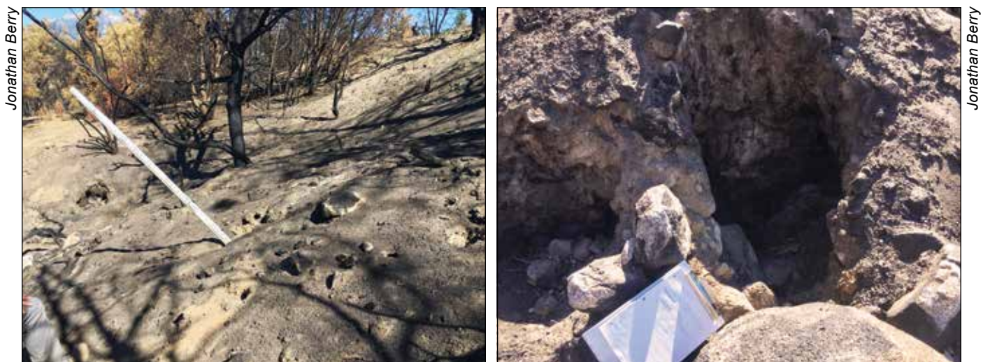
Figure 4.75—An earthen embankment of a dam where wildfire has burned the vegetation and tree roots, leaving deep voids in the embankment. Fire increases the risk of piping and dam failure.
