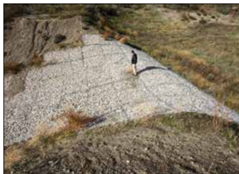
Figure 4.35—Existing undersized culvert fitted with an armored overflow dip to pass water without stream diversion or washing out the fill (a). Lower figures (b and c) show a stream diversion where a plugged culvert crossing sends water down the road rather than staying in its natural channel, causing considerable offsite damage. The bottom photos show a gabion mattress and turf reinforcing mats used to protect an embankment against overflow damage. (Figure adapted from Furniss et al. [1997])
