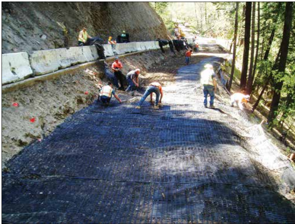
Figure 4.64—Cross section and installation of a typical deep-patch road-embankment repair. (Figure from Keller et al. [2011])
