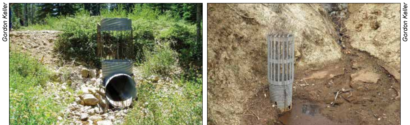
Figure 4.39—Two different designs of trash racks added to culverts in areas where wildfires occurred.
