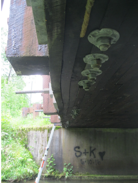
Figure 13 Hoffman Run outer lamination waviness
