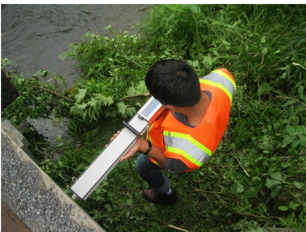
Figure 3 Resistance micro-drill in use at outer deck laminations.
