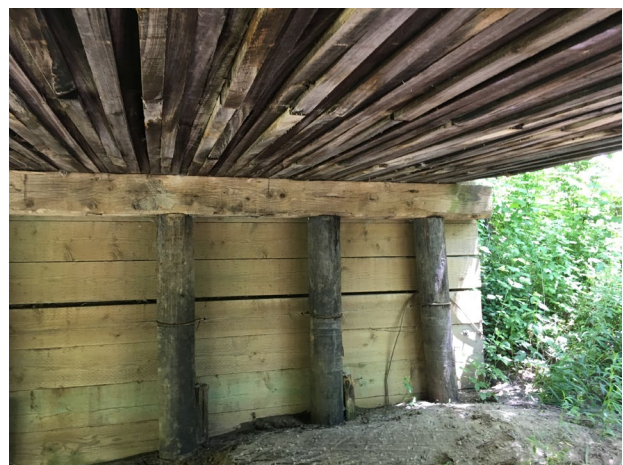
Figure 7 Hibbsville deck underside
