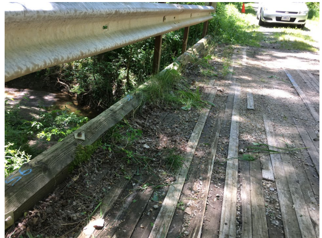
Figure 11 Hibbsville curb line vegetation
