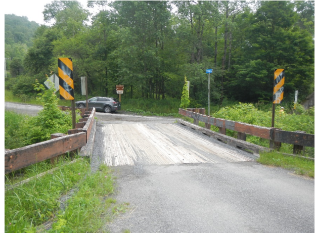
Figure 6 Hoffman Run stress-lam bridge.
