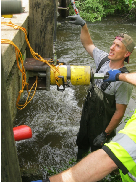
Figure 2 Jacking assembly showing the steel hardware and hydraulic equipment installed at one bar location.
