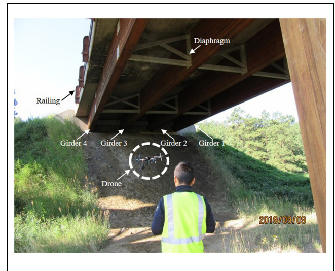
Figure 2. Three-span timber girder bridge located in Keystone, South Dakota.
