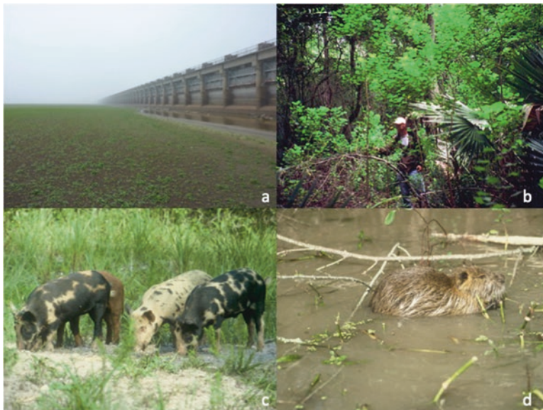
Fig. 6.4 Hydrological controls and invasive species are altering bottomland hardwood forests: (a) the Morganza Spillway in central Louisiana is part of an integrated system to control annual flooding and river movement (photo Sammy King); (b) invasive Chinese tallow grows rapidly in canopy gaps (photo Loretta Battaglia); (c) wild hogs are increasingly abundant; their rooting can negatively affect regeneration of native, large-seeded oaks and hickories (photo William Conner), and; (d) nutria are rodents from South America, now established in this system, where they occasionally cause “eat-outs” (photo William Conner)
