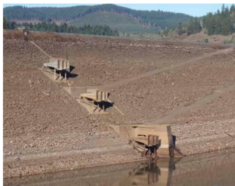
Drained Fall Creek Reservoir with “fish horn” outlets designed to allow juvenile salmon to migrate downstream when the reservoir is filled. Photo by Christina Murphy, Oregon State University.
