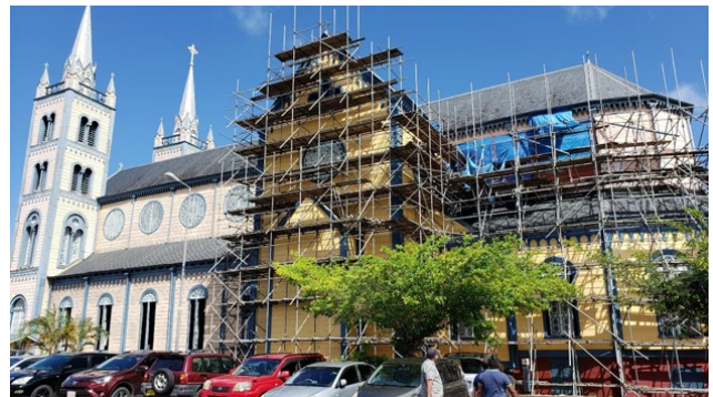
Figure 11—Exterior renovation of the Cathedral at the time of visit. Siding and external window joinery were being replaced.
