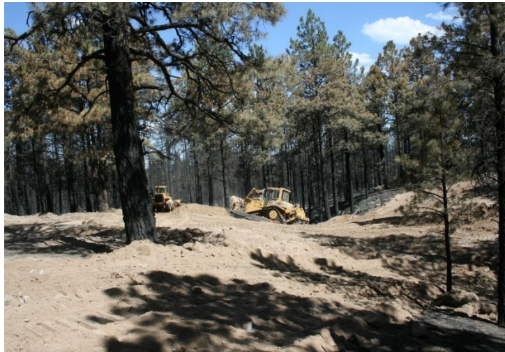
Figure 19. Culvert removal and low-water crossing construction on the Schultz Pass Road after the 2010 Schultz Fire, Coconino National Forest, Arizona (Photo courtesy of Dick Fleishman, Coconino National Forest)
