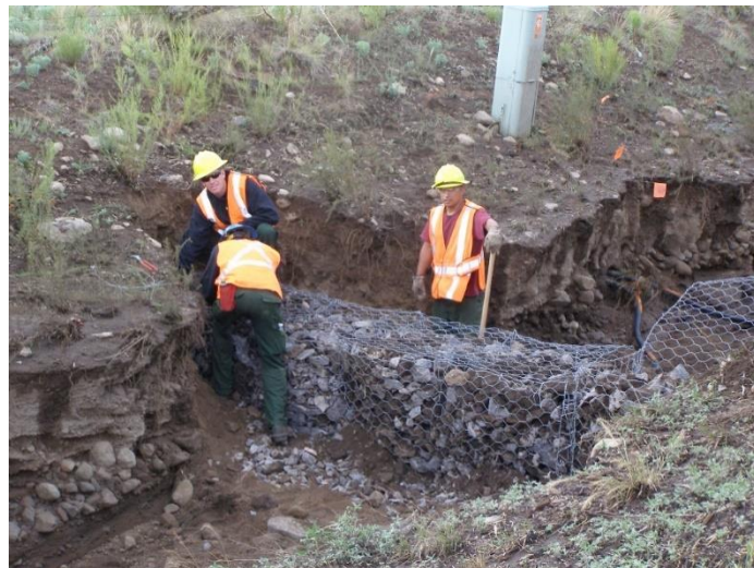
Figure 15. Construction of rock-wire gabions in the Campbell Avenue ditch after the 2010 Schultz Fire, Coconino National Forest, Arizona. (Photo by Daniel G. Neary, USDA Forest Service).
