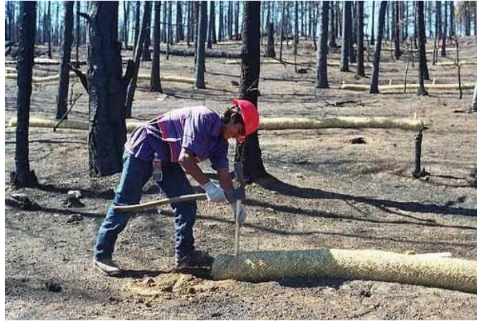
Figure 21. Straw wattles deployed on low gradient slopes to trap sediment in runoff. (Photo courtesy of the USDA Forest Service).
