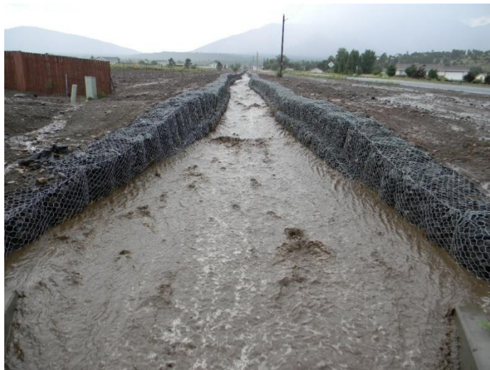
Figure 17. Second attempt at stabilizing the Campbell Avenue ditch using rock-wire gabions to stabilize the banks. (Photo by Daniel G. Neary, USDA Forest Service).
