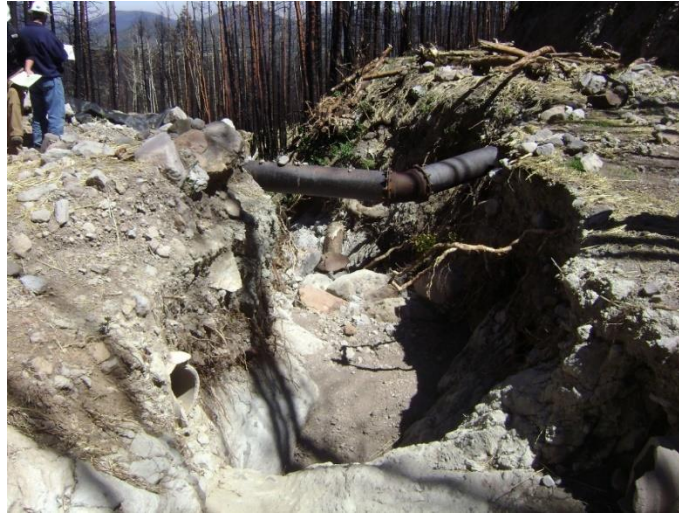
Figure 10. Major gully development after the initial rain event on the Schultz Fire, 2010, Coconino National Forest, Arizona, USA. (Photo by Daniel G. Neary, USDA Forest Service).
