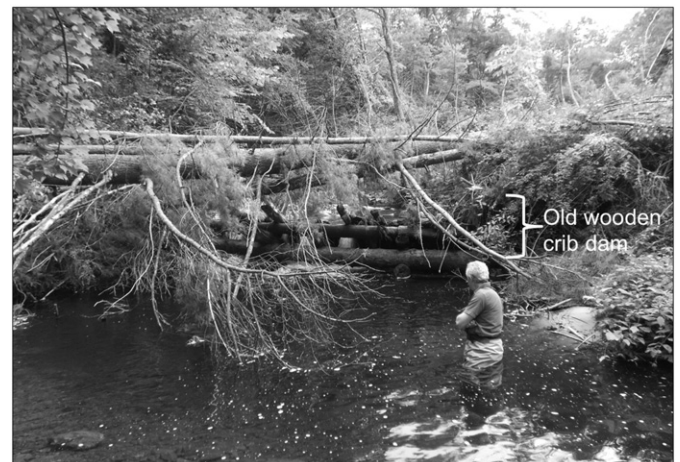
Fig. 12. Exhumed wooden crib dam. Photo taken soon following the 28 June 2013 flood.
