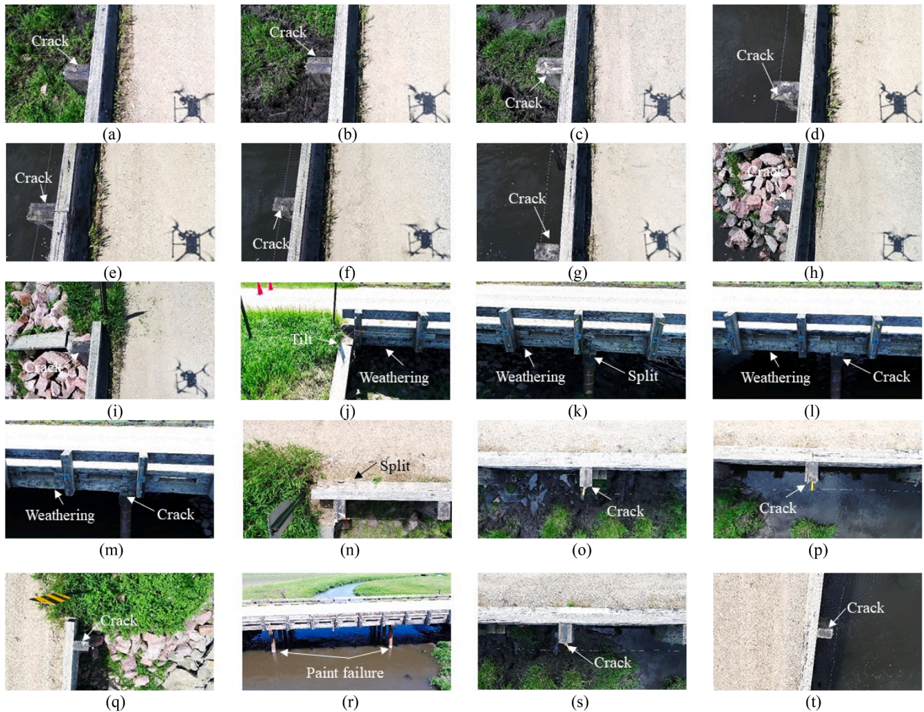
Fig. 14. Optimized UAV inspection images adjusted with the brightness of 20%, contrast of 20%, and sharpness of 30%: (a) crack on the railing on SS1; (b) crack on the railing on SS1; (c) crack on the railing on SS3; (d) crack on the railing on SS3; (e) crack on the railing on SS5; (f) crack on the railing on SS5; (g) crack on the railing on SS5; (h) crack on the railing on SS7; (i) crack on the railing on SS7; (j) tilt and weathering on NS1; (k) weathering and split on NS3; (l) weathering and crack on NS3; (m) weathering and crack on NS7; (n) split on NS1; (o) crack on the railing on SS1; (p) crack on the railing on NS1; (q) crack on the railing on NS7; (r) paint failure on NS; (s) crack on the railing on NS5; and (t) crack on the railing on NS5.
