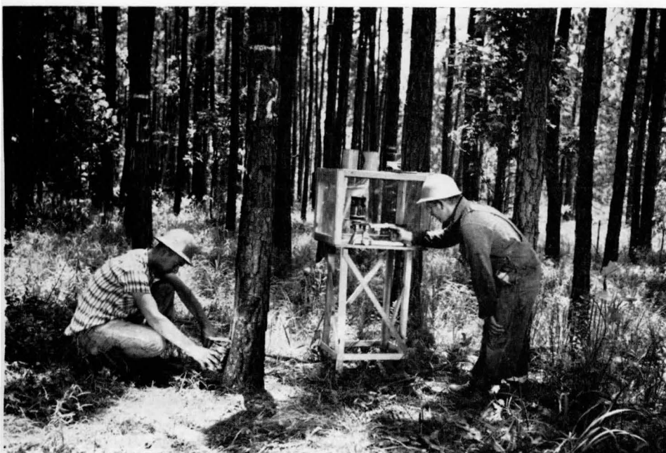
Larry Gillespie (left) takes a can from one of the test trees to weigh collected gum while Hansford Ray weighs the 2-week yield of another micro-chipped slash pine in the experiment.
