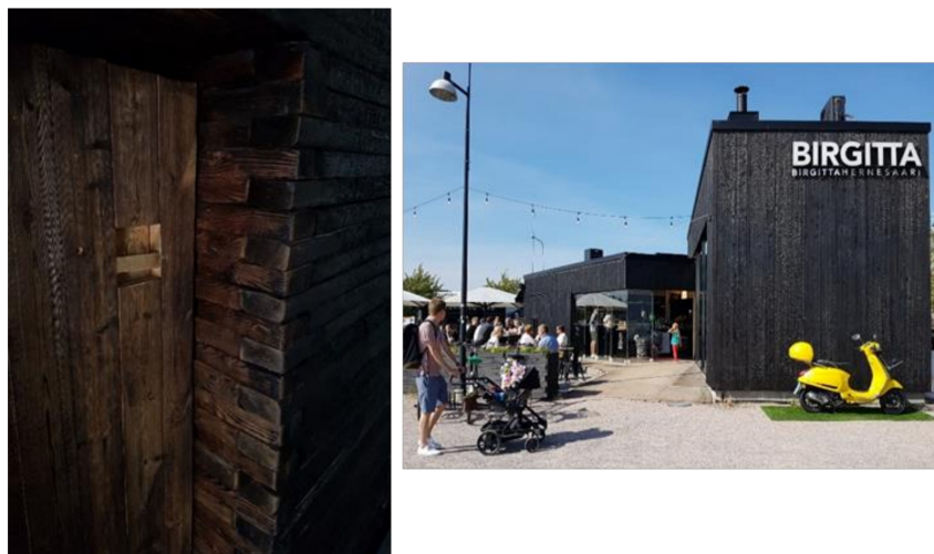
Figure 4. A detail of a sauna made from surface charred elements in Espoo, Finland; a restaurant in Helsinki with a flame charred exterior.
