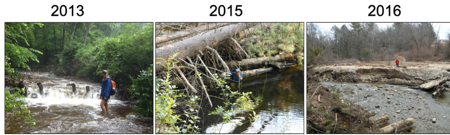
Fig. 11. Photo of wooden crib dam over time. Pelham Dam was removed in fall of 2012 and the upstream knickpoint migration exhumed the previously unknown undated (ca. 1780?) wooden crib dam. Middle photo (2015) shows deep plunge pool that remained until subsequent removal of wooden crib in December 2016.
