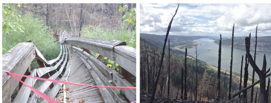
Figure 2. The Eagle Creek fire (2017) closed many trails in the Columbia River Gorge National Scenic Area. The fire resulted in damaged recreational infrastructure (bridge on left), and the severity of the fire affected the scenic value of the area (right). Trails remain closed at the time of writing, 3.5 years after the fire. Source: USDA Forest Service.
