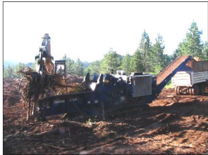
Fig. 2. Landing for the wood chipping process in the biomass impacts study at the New Meadows, Idaho site.
