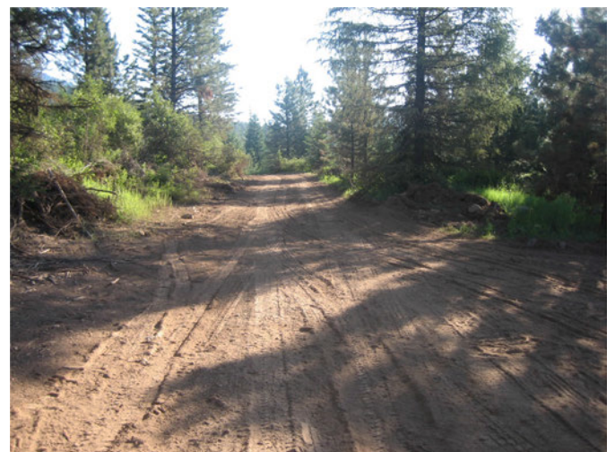
Fig. 10. Pulverized road condition at the New Meadows, Idaho site for the biomass utilization impacts study in the NW U.S.
