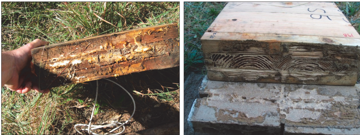
Figure 5. Examples of fungal decay (left) and termite damage (right) to 3-ply Douglas-fir CLT in a covered ground proximity test after four years.
