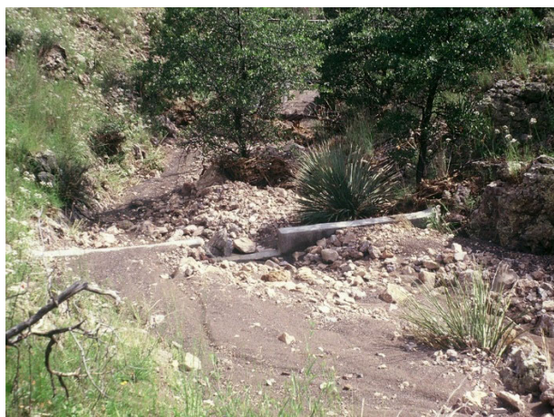
Figure 9. A sediment basin was located above the flumes on each of the Cascabel Watersheds to accumulate sediment that is deposited near the outlets of the watersheds. (Photo by Daniel Neary, USDA Forest Service).
