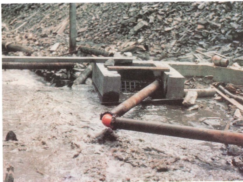
Figure 2.--High water heavily laden with mine tailings bypassing the coffer dam on Blackbird Creek (May 1967).
