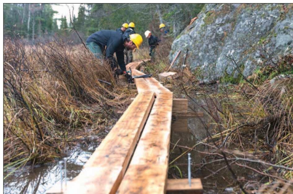
Nature Conservancy staff and volunteers build the boardwalk. Photo by Creative Fauna.
