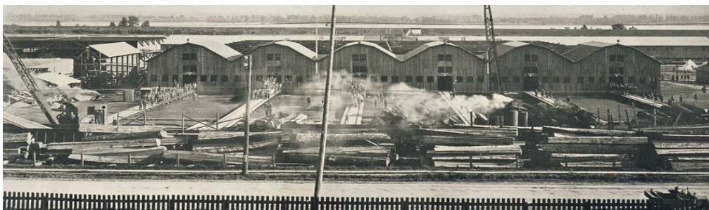
Figure 9—Built in 1917, the spruce mill at Vancouver Barracks (Vancouver, Washington, USA) was the largest of its kind in the world and was responsible for the production of millions of board feet of lumber specifically for aircraft production (National Park Service photo).
