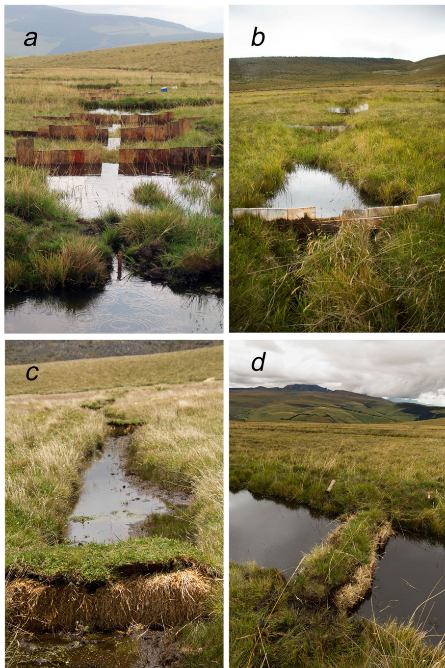
Fig. 5 Examples of the barriers constructed with wood planks ( a and b ) or straw bales ( c and d ) to slow down water movement along the ditches, and promote rewetting in the Chakana peatland
