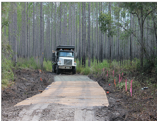
Figure 30—A section of a low-volume road reinforced with mats at the Apalachicola National Forest.
