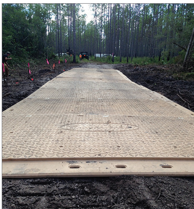
Figure 28—High-density polyethylene mats (HDPE) are designed to reinforce existing soils, providing support for vehicular and pedestrian traffic and potentially providing a foundation for heavy equipment or temporary buildings.
