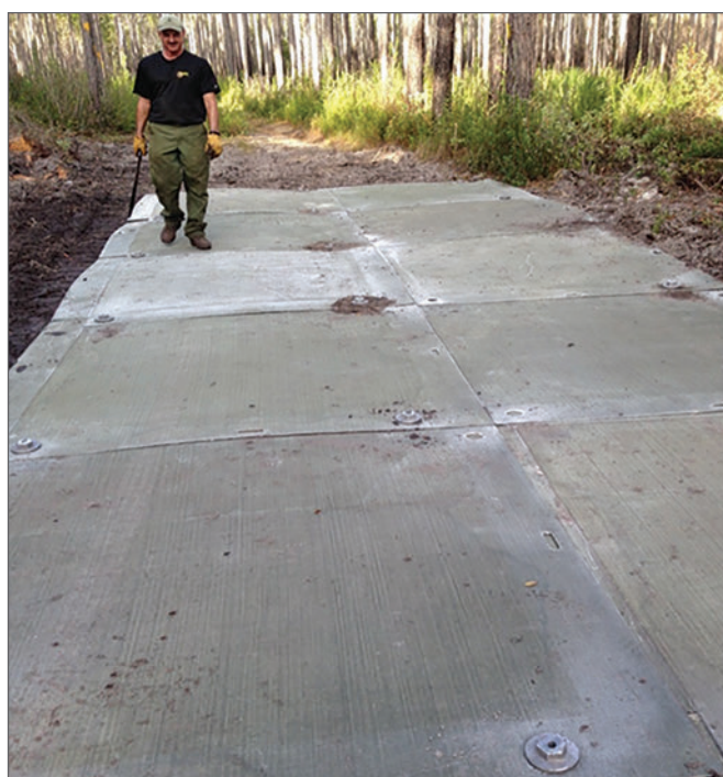
Figure 29—The United States Government designed this mat using thin panels.
