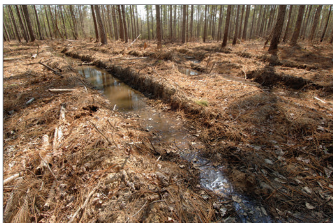
Figure 6—During the rainy season, ruts become preferential flow paths and result in erosion.
