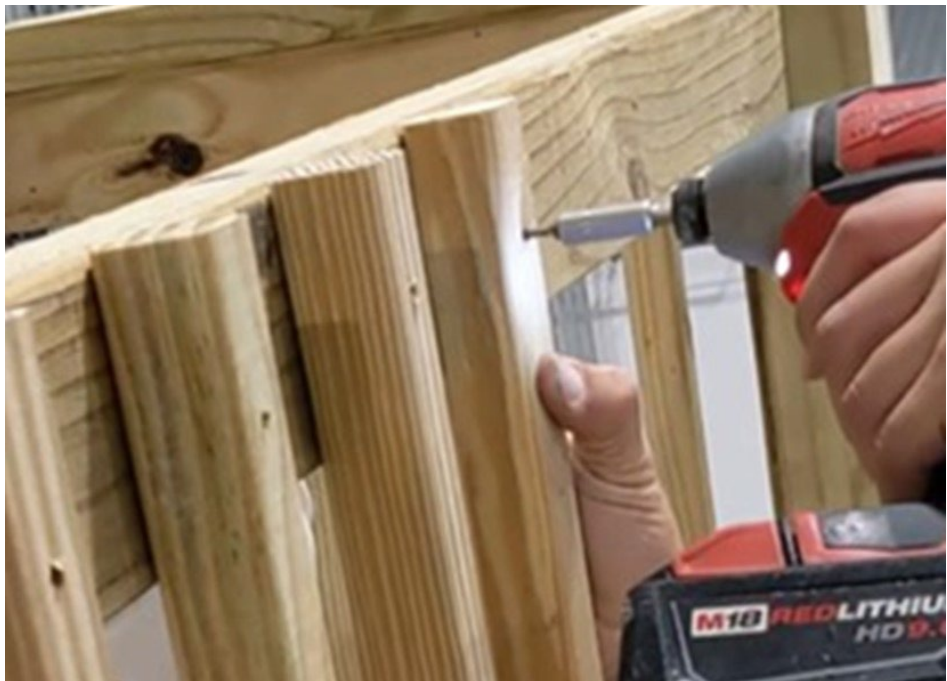
Figure 73. Install Spindles in Rail System
