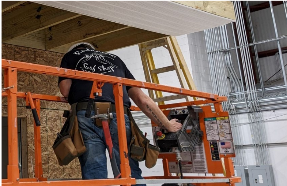
Figure 62. Install Perforated Soffit Panels
