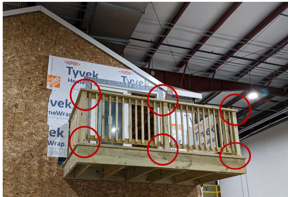
Figure 79. Inspect All Wood Railing Components
