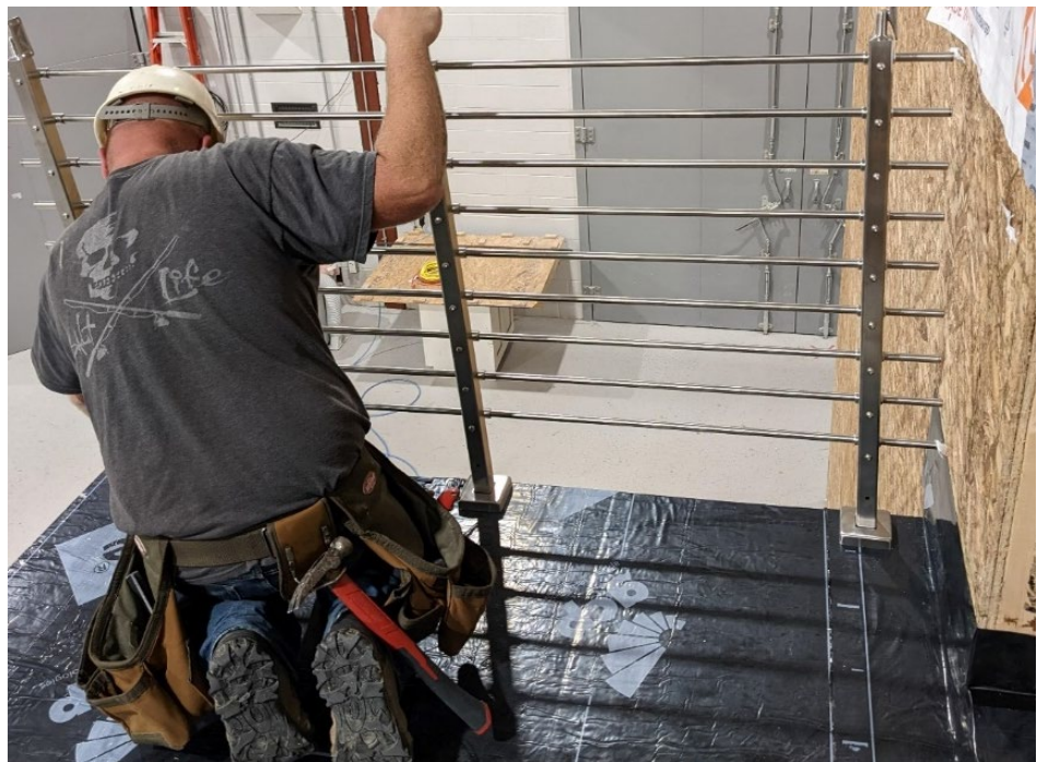
Figure 56. Install Metal Railing System
