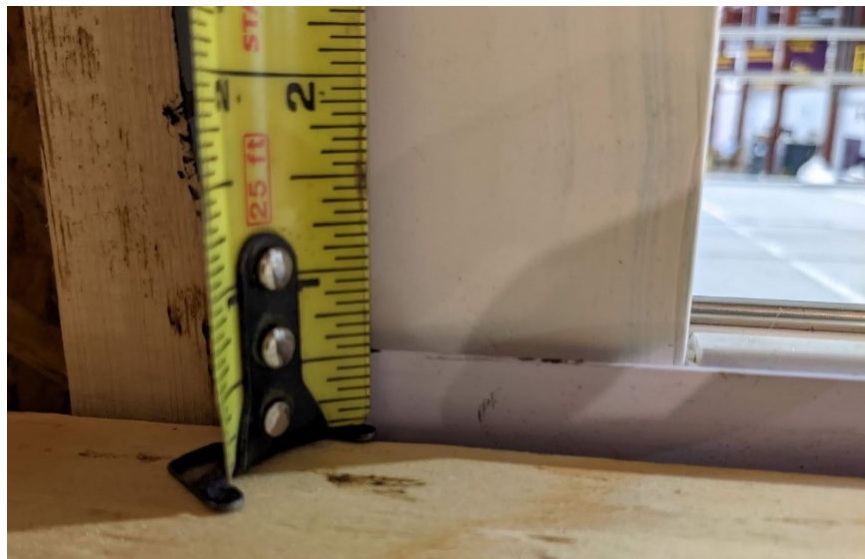
Figure 61. Measure Height of Threshold for Accessibility
