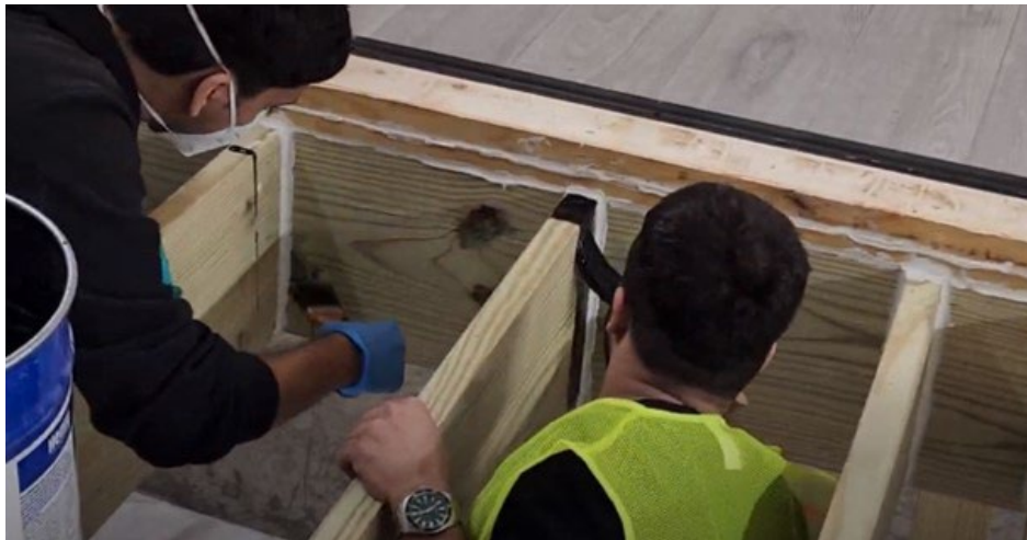
Figure 66. Seal Intersection with Liquid-Applied Flashing
