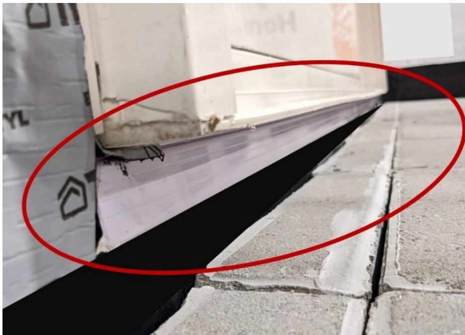
Figure 77. Inspect Exterior Door Threshold
