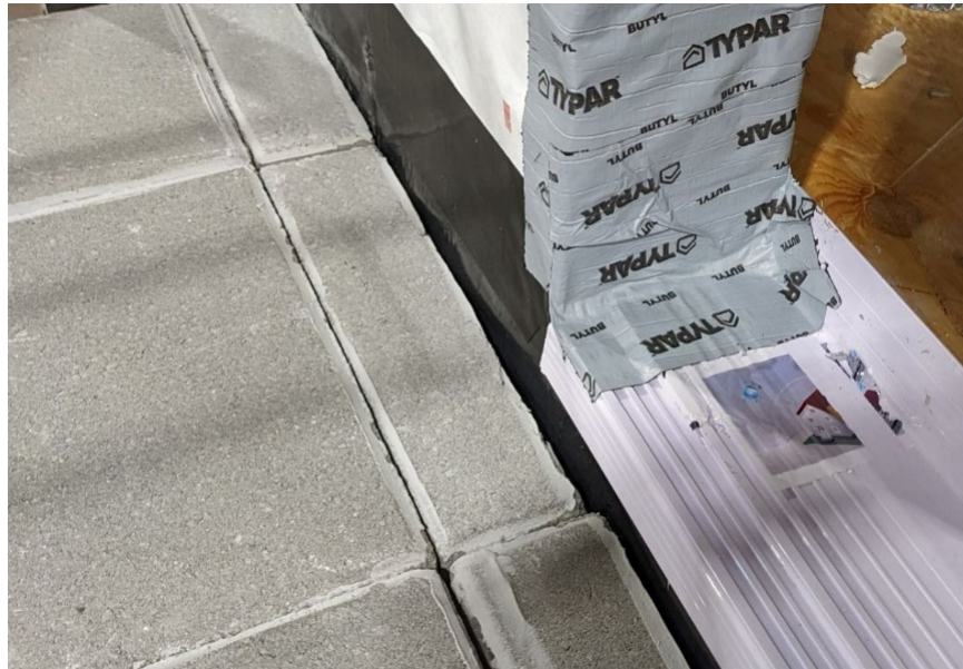
Figure 60. Install Pan Flashing at Threshold
