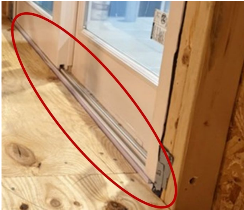
Figure 76. Inspect Interior Door Threshold
