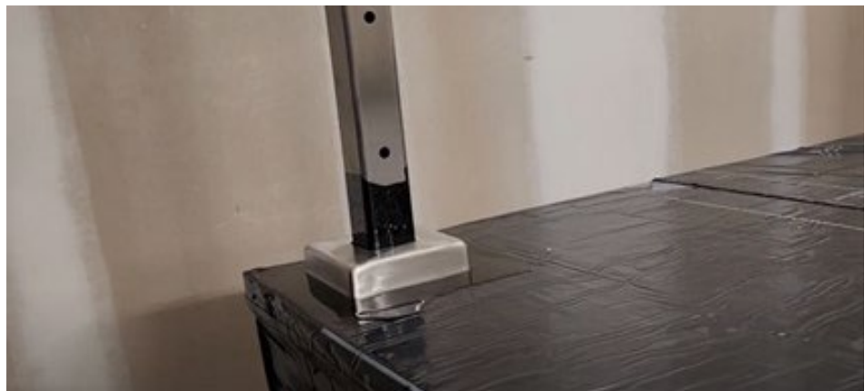
Figure 55. Install Rail Post Cover
