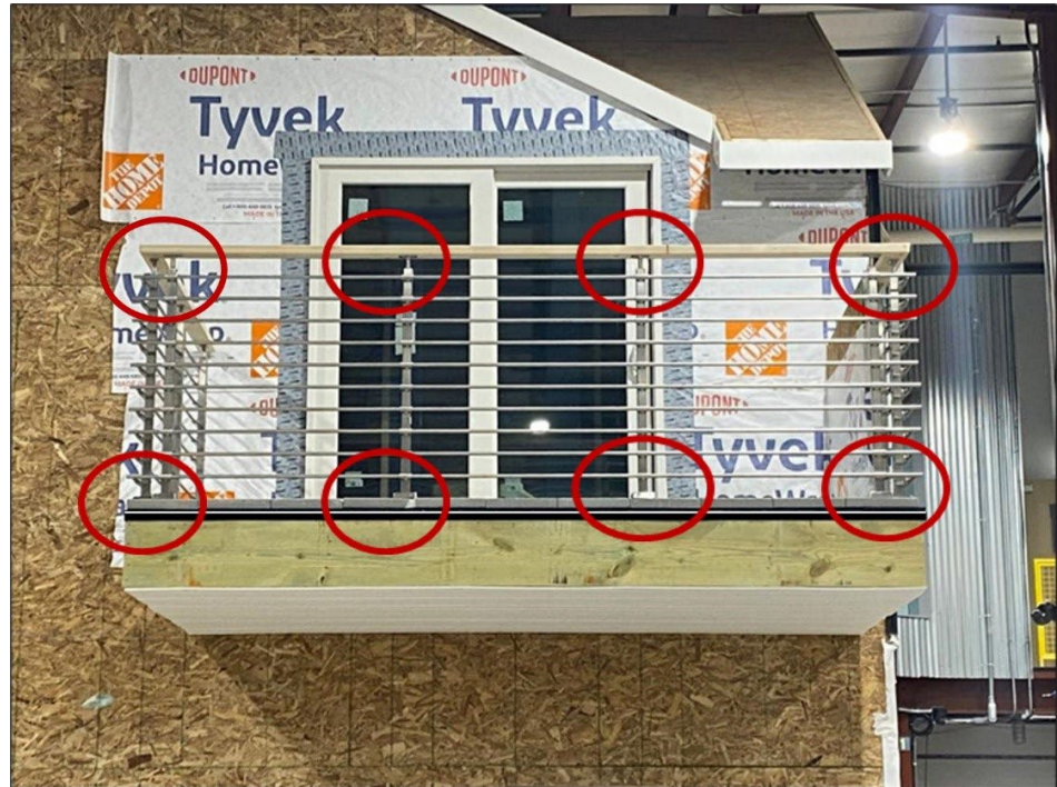
Figure 78. Inspect All Metal Railing Components
