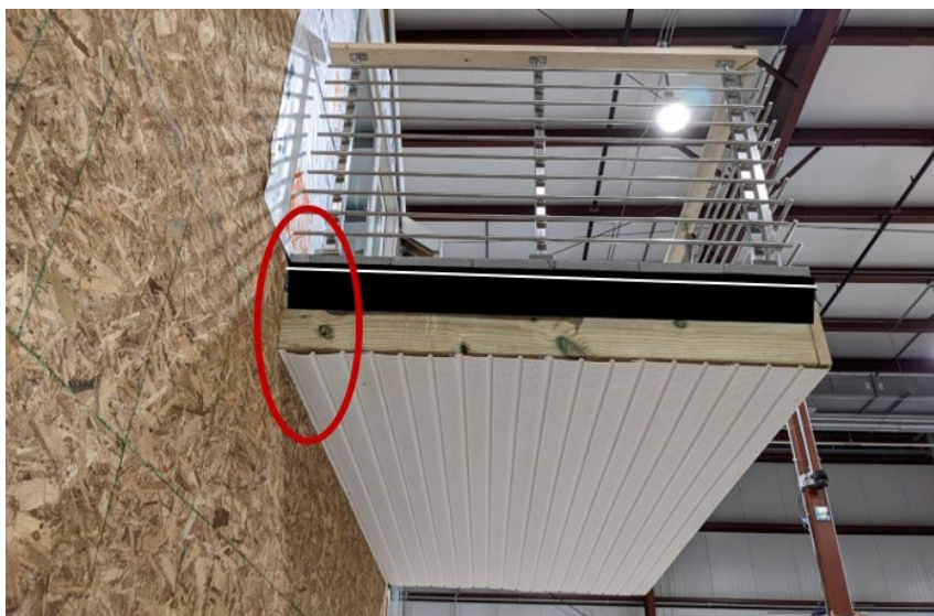
Figure 75. Inspect Intersection Between Wall and Structure Members
