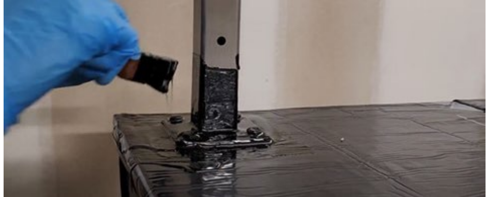
Figure 54. Seal with Liquid-Applied Flashing
