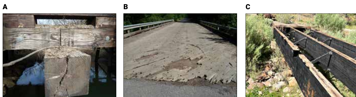
FIGURE 2. Premature breaking of the preservative barrier resulting in incipient decay caused by: (a) mechanical damage, (b) weathering damage, (c) fire damage (Lebow, 2022).
