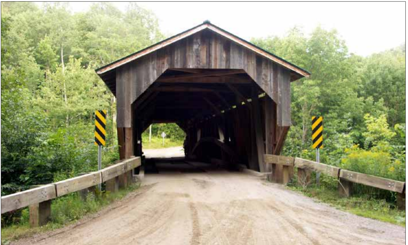
FIGURE 3. Grist Mill Covered Bridge, Lamoille County, Vermont (Bridge Hunter, 2022).
