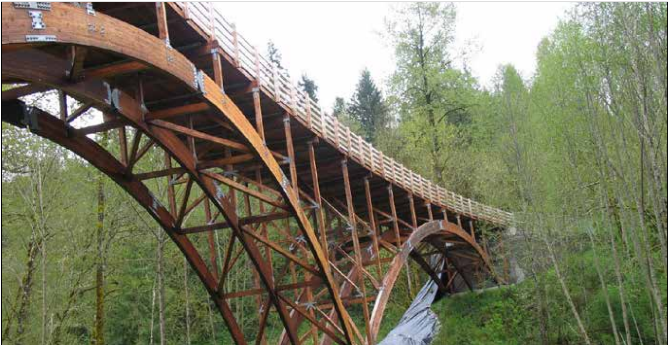
FIGURE 3. The Lower Burnett Road Bridge in Buckley, Washington (Turner, 2010).
