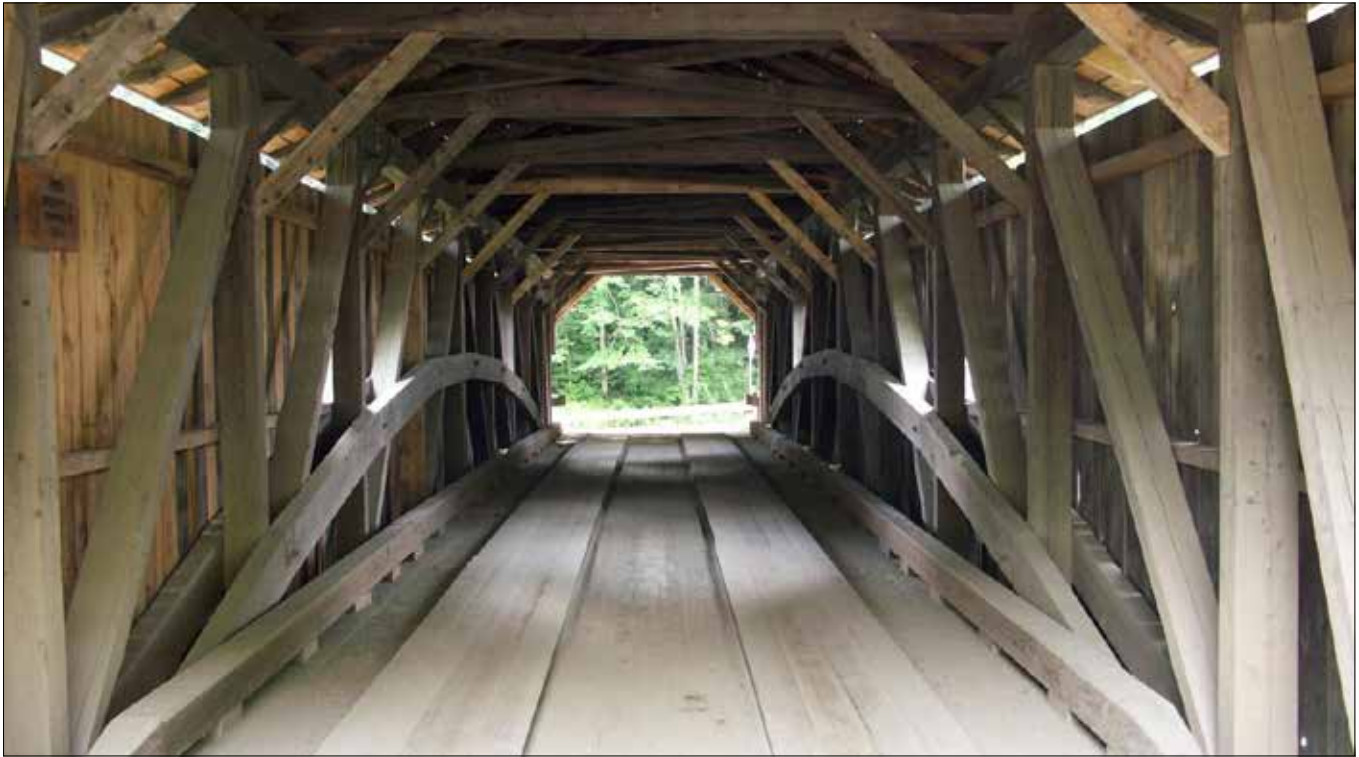
FIGURE 3. Grist Mill Covered Bridge, Lamoille County, Vermont (Bridge Hunter, 2022).
