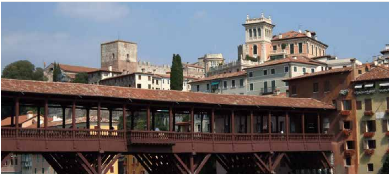
FIGURE 1. Example of trestle and roofed beam bridge (Porta, 2019).
