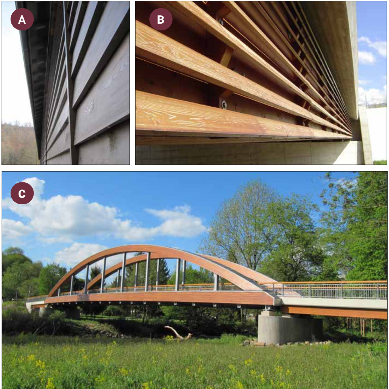
FIGURE 4. Side cladding for efficient timber bridge design in (a) Germany, (b) Switzerland, and arch girders protected by stainless steel flashing plates (c) in Germany (Simon and Koch, 2016).
