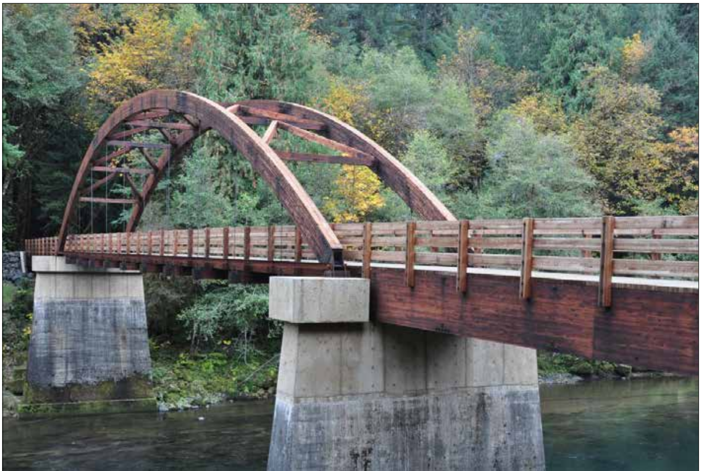
FIGURE 6. Tioga Bridge over the North Umpqua River in Oregon (Bridge Hunter, 2022b).
