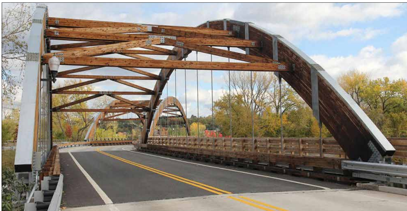
FIGURE 4. Overpeck Park Bridges in Teaneck, New Jersey (Bridge Hunter, 2022a).
