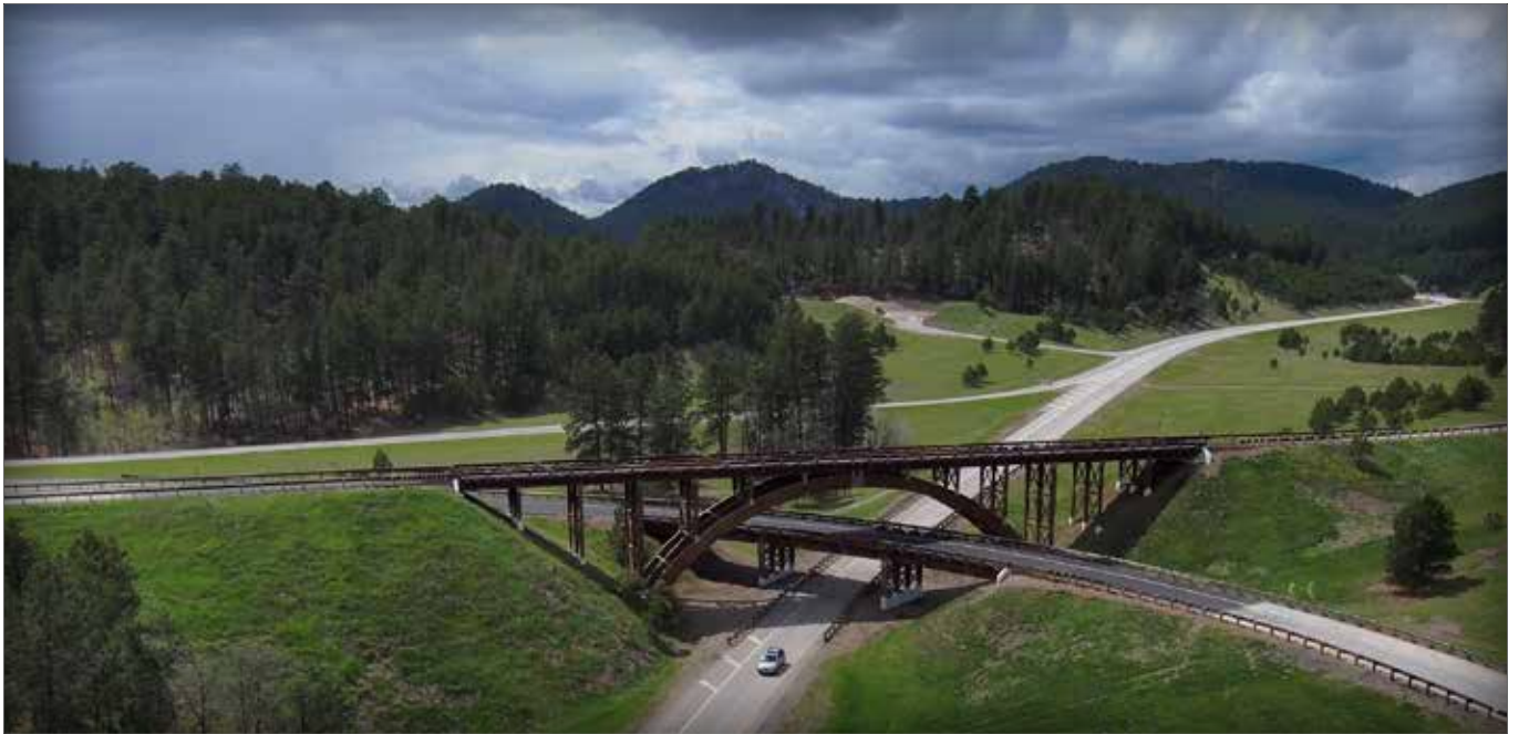
FIGURE 1. Keystone Wye bridge built in 1968 in South Dakota (South Dakota Department of Transportation, 2022).
