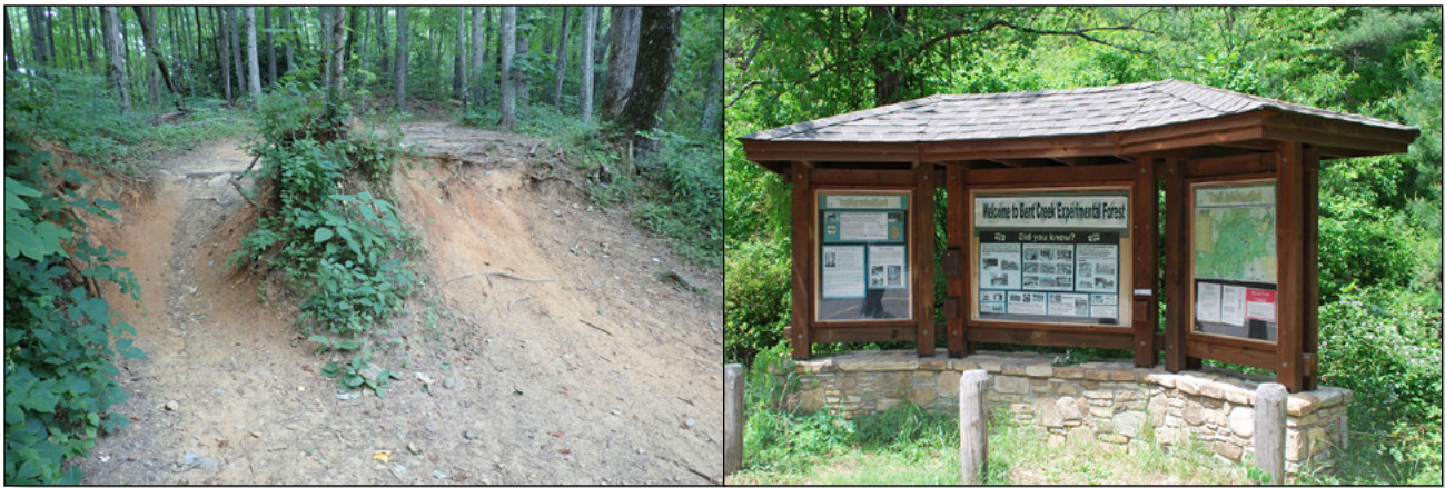
LEFT: Soil erosion from bike traffic on an illegal, user-created trail; RIGHT: Bent Creek kiosk at low-elevation entrance.
