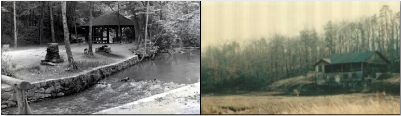
LEFT: Bent Creek campground pavillion, approximately 1942; RIGHT: Lodge at drained Deer Lake, approximately 1980.
