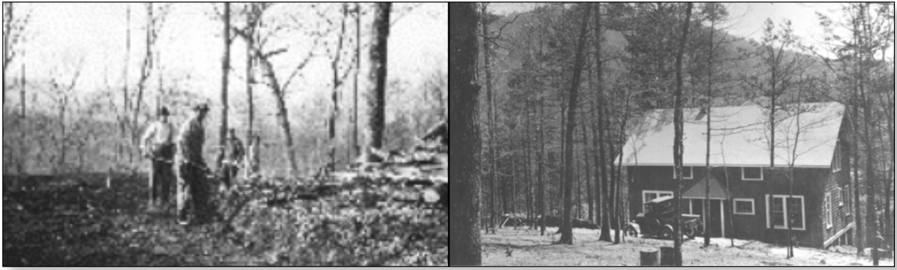
LEFT: Work crew building Hard Times Road; RIGHT: The small building that served as the original 1925 laboratory/office at Bent Creek.
