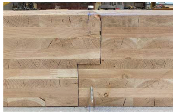
Figure 4 Shiplap Connection used for Longitudinal Panel Deck
