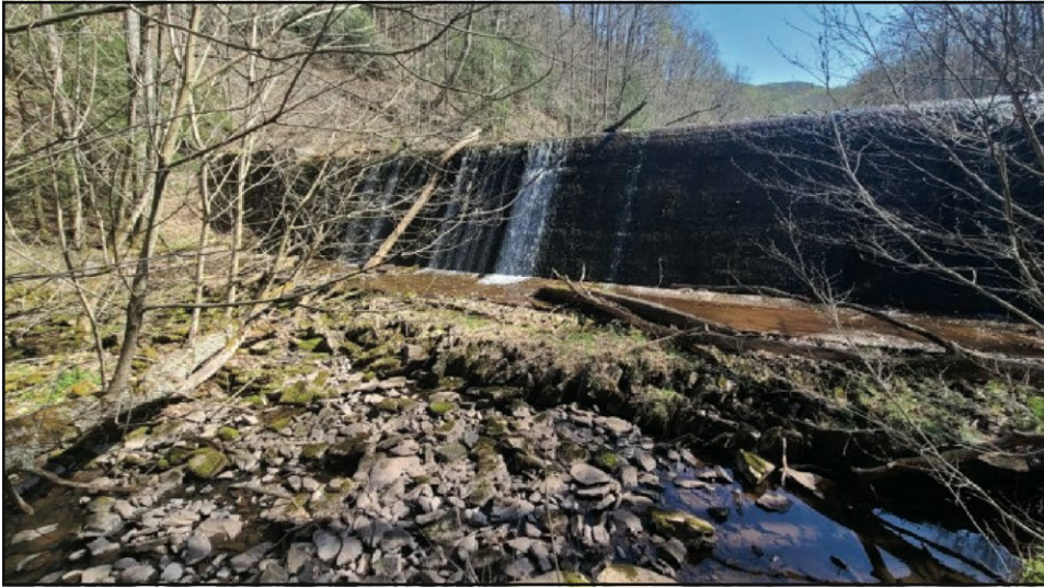
Figure 11. Photo of Parsons Dam on Ellick Run facing southeast.
