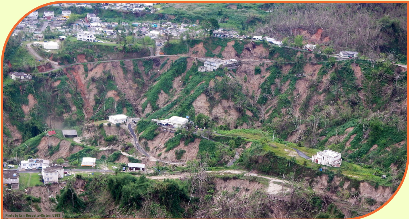
Landslide damage after Hurricane Maria. Utuado, Puerto Rico, 2017. Almost 60% of trees lost branches, snapped in half, or were uprooted.
