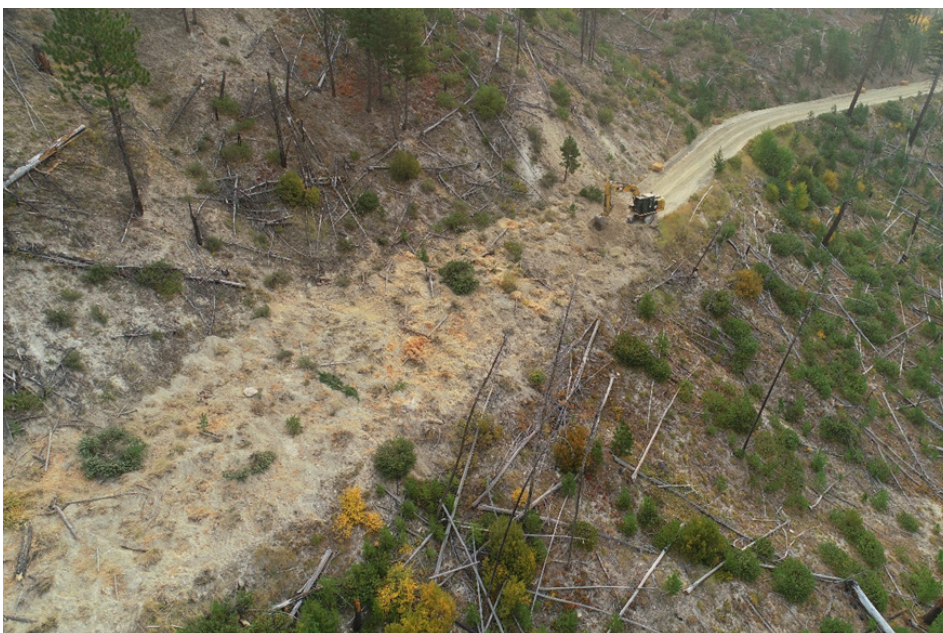
Figure 5: Road decommissioning by fully recontouring an unstable road above critical salmon spawning habitat in the Dollar Creek drainage of the Boise National Forest. Image thanks to USFS GTAC/ Red Castle Resources.
