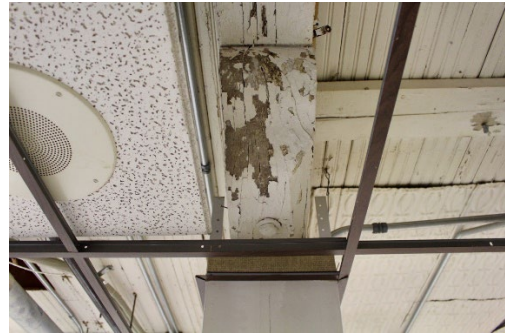
Figure 12—Room 02305. Member shifting off-center.
