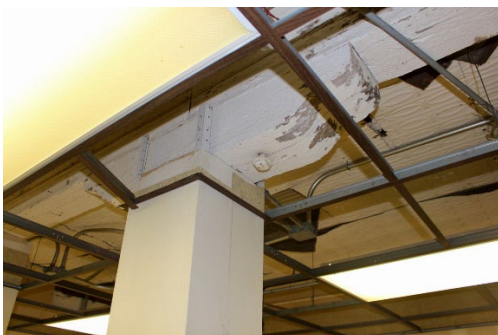
Figure 11—Room 02305. Note that bolt is not in contact with the timber member.
