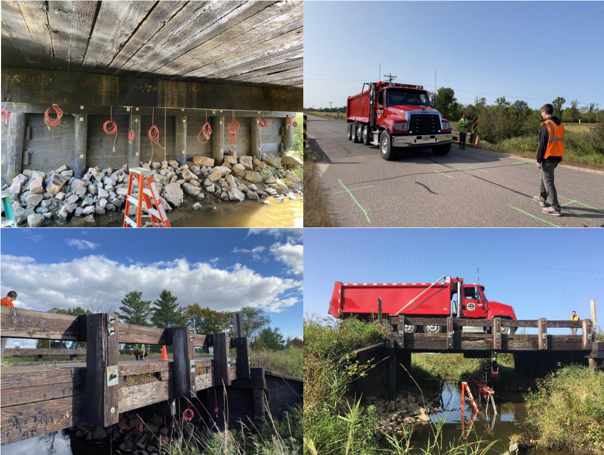
Figure A. 1 Bridge photos for B030174
