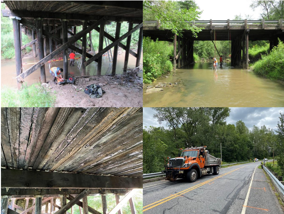
Figure A. 4 Bridge photos for P320083
