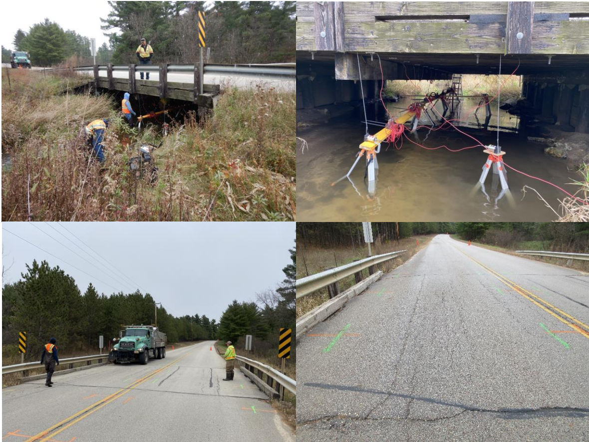
Figure A. 8 Bridge photos for P410953
