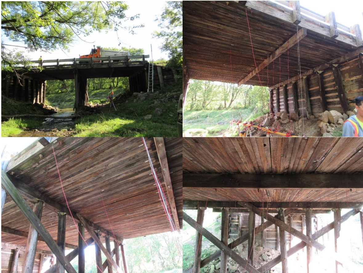
Figure A. 5 Bridge photos for P320110
