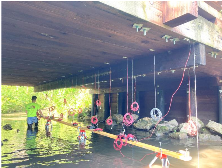
Figure 4-49 Sauk County Bridge B560224 Spreader Beam
