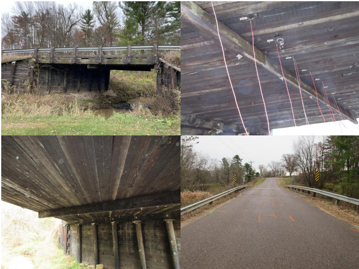
Figure A. 6 Bridge photos for P410140
