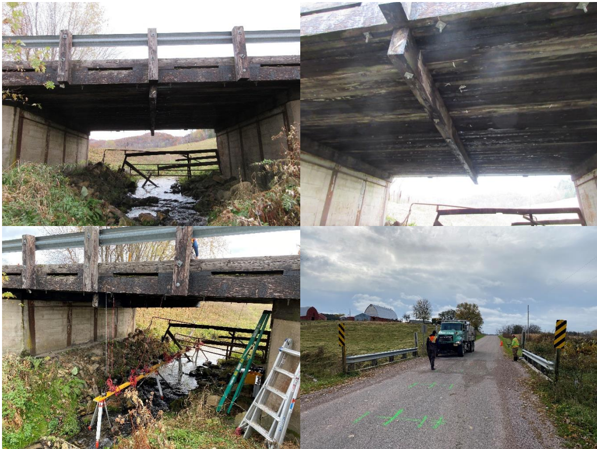
Figure A. 7 Bridge photos for P410923
