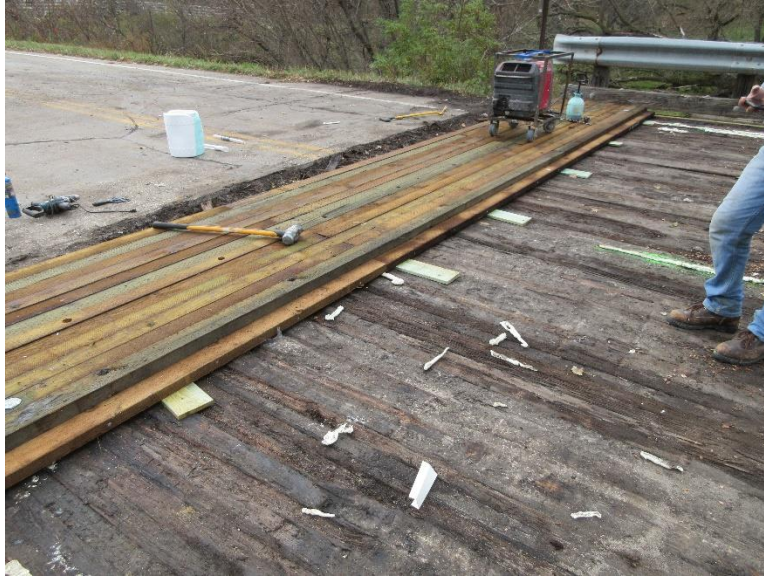
Figure 4-35 Transverse Timber Slab Retrofit under Construction
