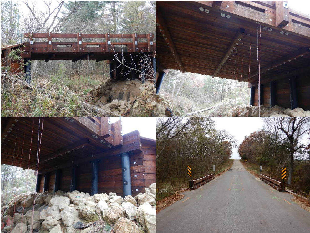
Figure A. 9 Bridge photos for B410315
