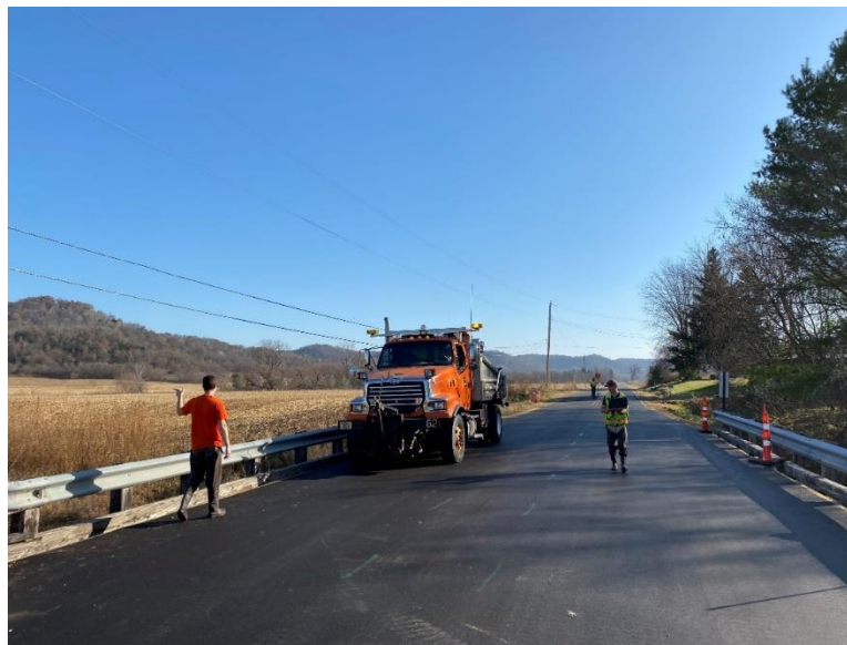
Figure 4-13 Load truck crossing the bridge
