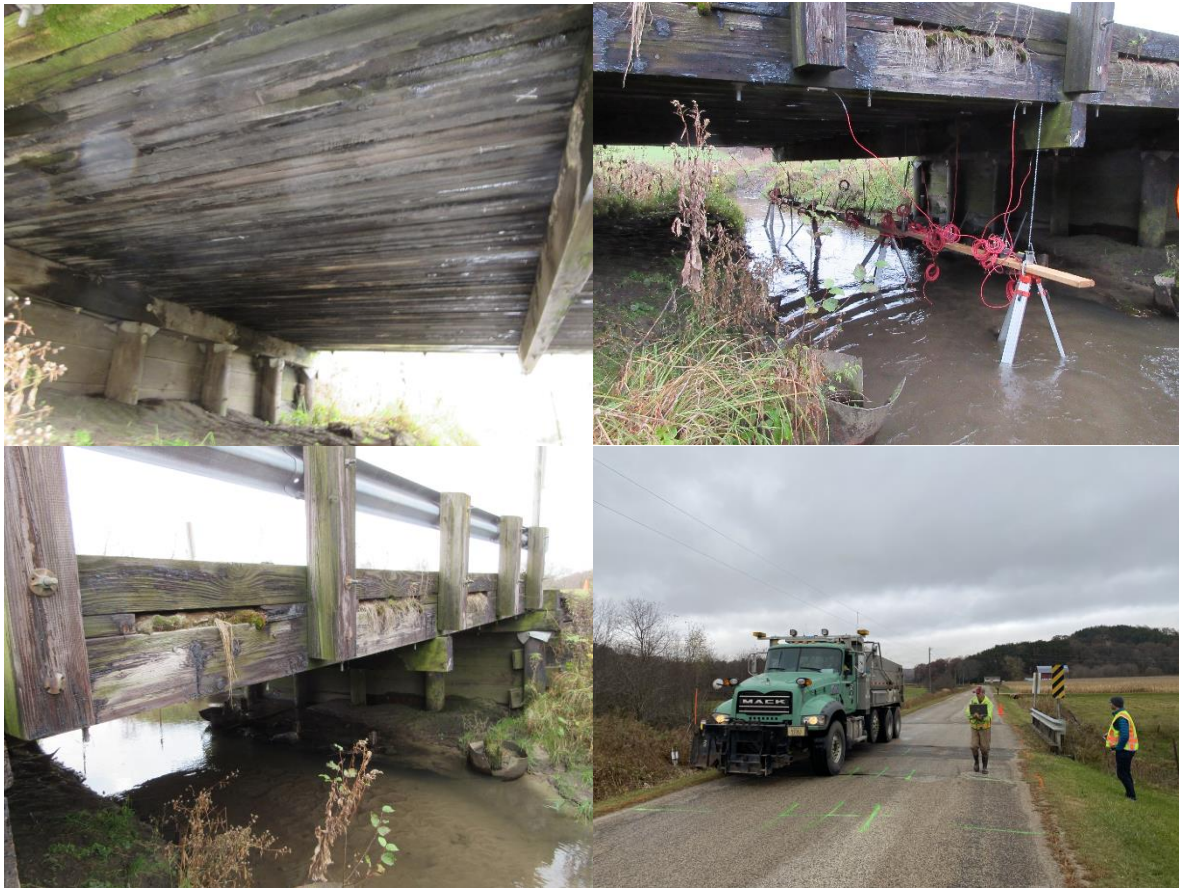
Figure A. 10 Bridge photos for P410948
