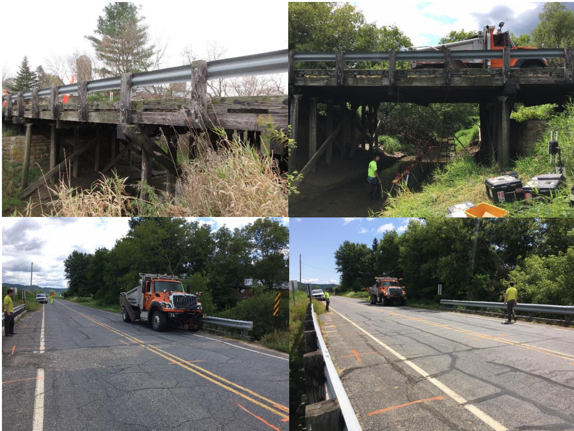
Figure A. 3 Bridge photos for P320064
