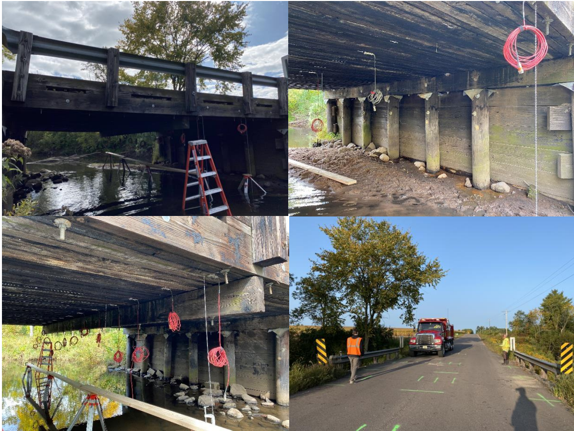
Figure A. 2 Bridge photos for P320079
