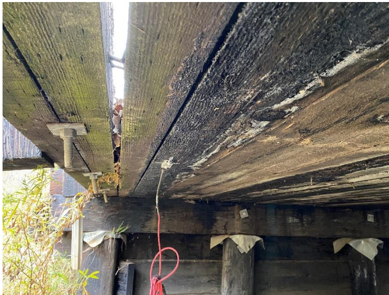
Figure 4-56 Delamination near edge of slab (Monroe Co. P410953)
