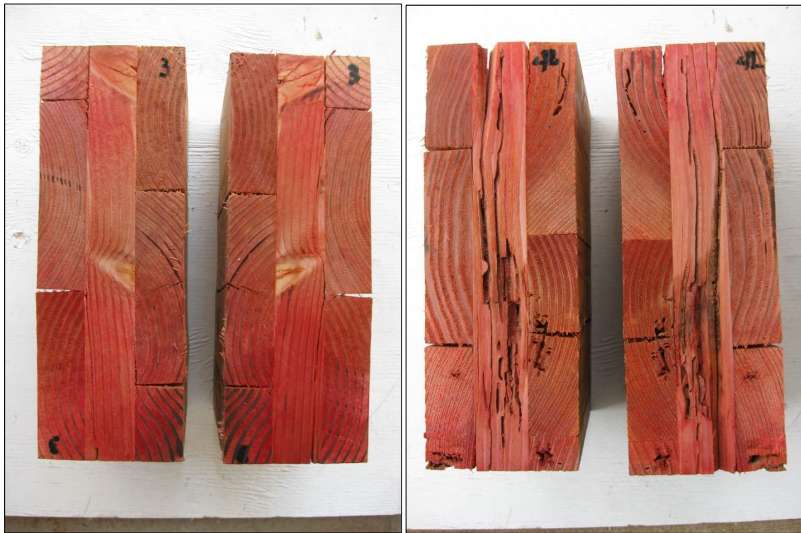
Figure 9: Cross-cut curcumin-stained samples treated with borates at test initiation (preventative) (left) after six years and remedial treatment (right) after five years showing boron diffusion (red) surrounding dormant termite galleries.
