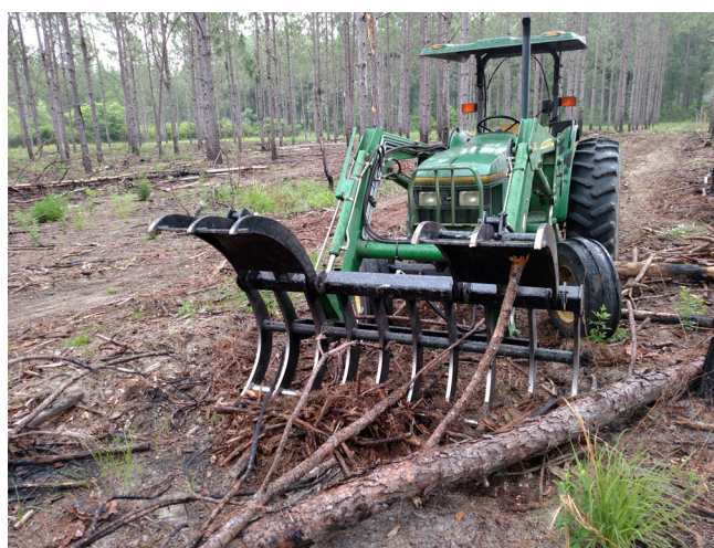
Figure 5—Removal of logging slash from plantations using a grapple rack. Photo taken in May 2015 after commercial thinning. (Photo courtesy of The Jones Center at Ichauway)
