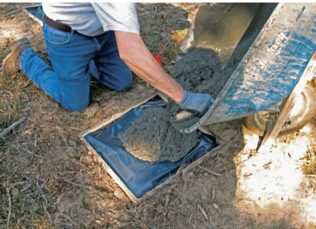
▲ Fig. 2. Concrete slab soil sample (no PVC) plot during concrete pouring at the HEF in 2023.
