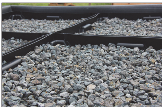
Figure 6. Blue roof trays with Stalite.
