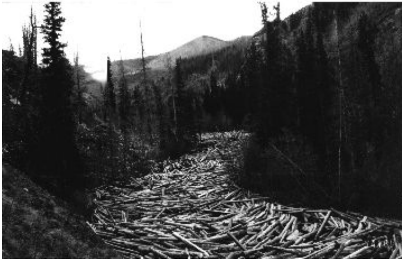
Figure 3.12 —Logs being floated down streams from the harvest site to mills. USDA Forest Service historic photo. Date and location unknown.
