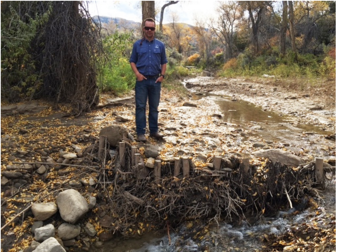
Figure 4.20 —A beaver dam analogue (BDA), created from posts pounded into the streambed and bank, on Miller Creek in central Utah. Channel aggradation is occurring 6 months after installation. Jordan Nielson, with Trout Unlimited, stands nearby. Courtesy photo by Allison Jones, Allison Jones LLC.
